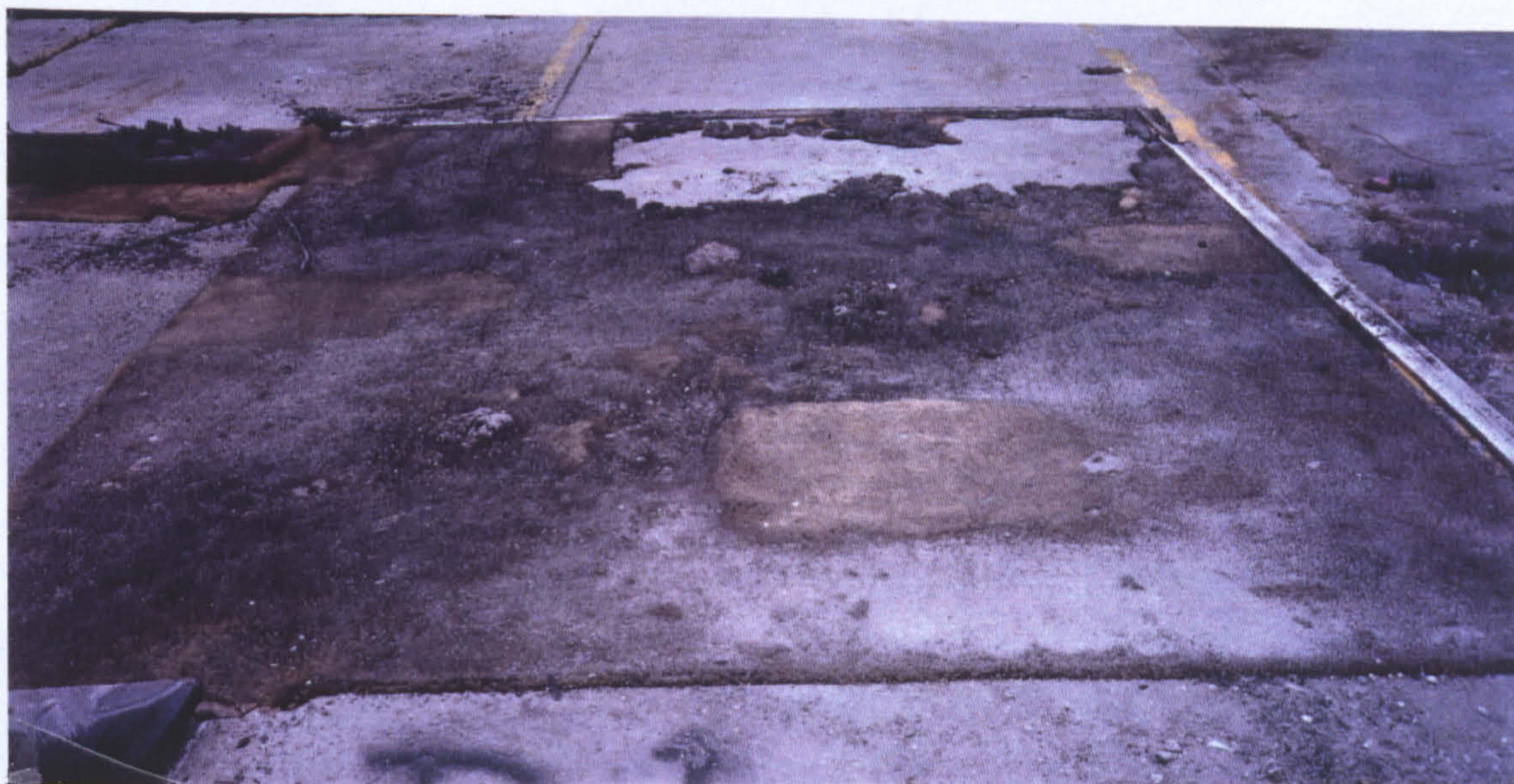
Fig. A3.10.4.15: The carpet from the same room test removed to make the burn patterns more visible. Localized deep charring in centre and left side were not produced by accelerant. The complete combustion of the carpet in the right rear corner was the result of the prolonged fire in the bed (which represented the primary fuel load in the room throughout much of the fire).
