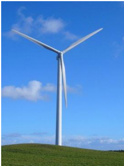
Figure 1-1: Danish concept, horizontal axis, three bladed wind turbine [1].
