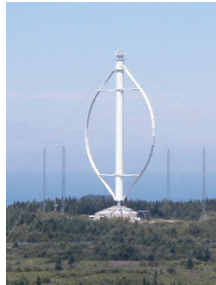
Figure 1-2: Vertical axis wind turbine [2].
