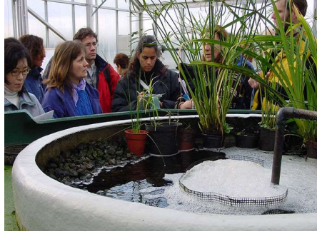
Figure 14 Natural Sewage Treatment Plant (Findhorn Foundation)
