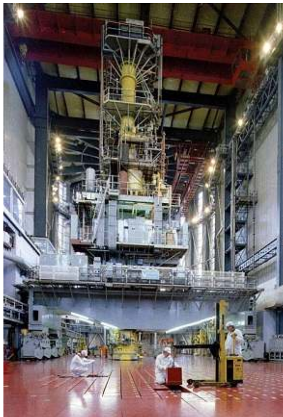
Figure 5.4: Dungeness B Refuelling Machine (Source: [92])
