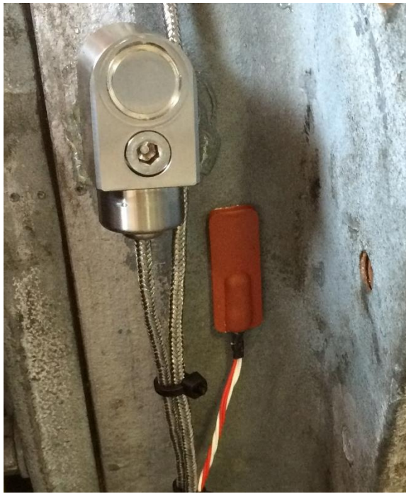
Figure 8: PT100 sensor (red patch) and accelerometer mounted on the main bearing
