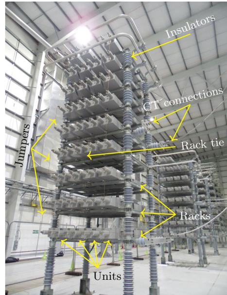
Figure 2.4: A large capacitor bank
