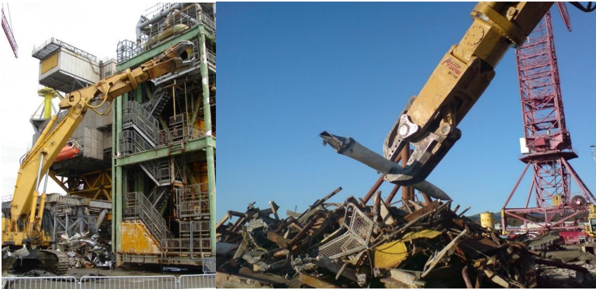
Figure 2. 9: MTR 160 S decommissioning a platform off the coast of Norway (Alligator, 2021)
