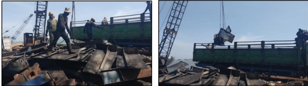
Figure 10. 10: Pictures of moving pieces of steels into the truck
