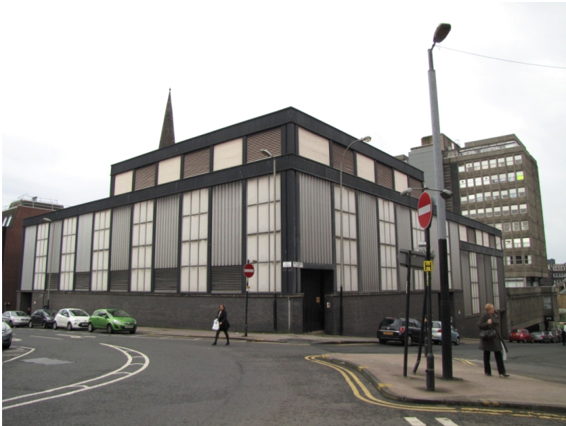
Figure 7.11: External view of the West George Street indoor substation.
