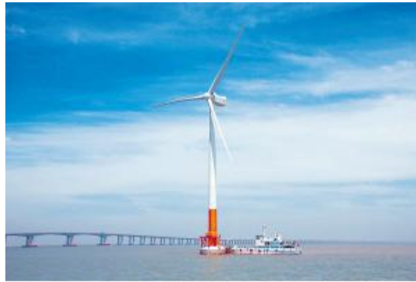
Figure 1.5 Donghai bridge offshore wind farm
