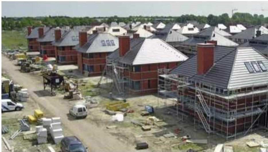
Figure 3 .34 Mass produced modules
