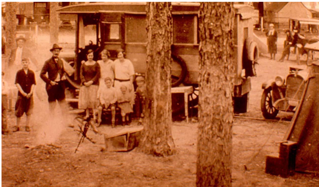
Figure 3 .16 Motorhome One of the first models of Motorhome in early 20 th century. Picture (Neff, 2010).
