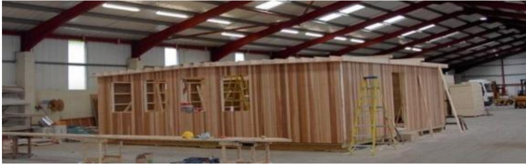
Figure 3 .33 Modular timber structure The whole unit can be built in the factory and then moved to the construction site. Picture (R. G. Stones, 2013).
