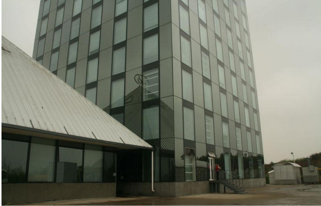
Figure 3 .69 T30, not an architectural gem
