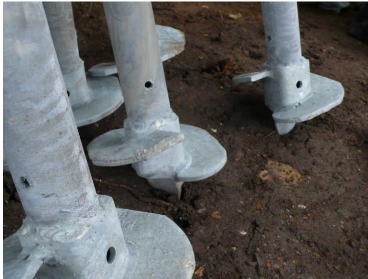
Figure 3 .74 The Hertfordshire house's foundation Screw Piles. Picture (Facit Homes-c).
