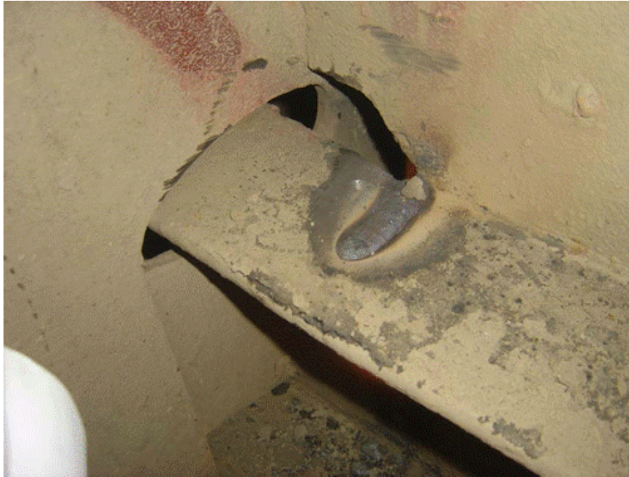
Figure 2.7 Material repairing at the inner mouse-hole location (WU Xiaoyuan, 2007)
