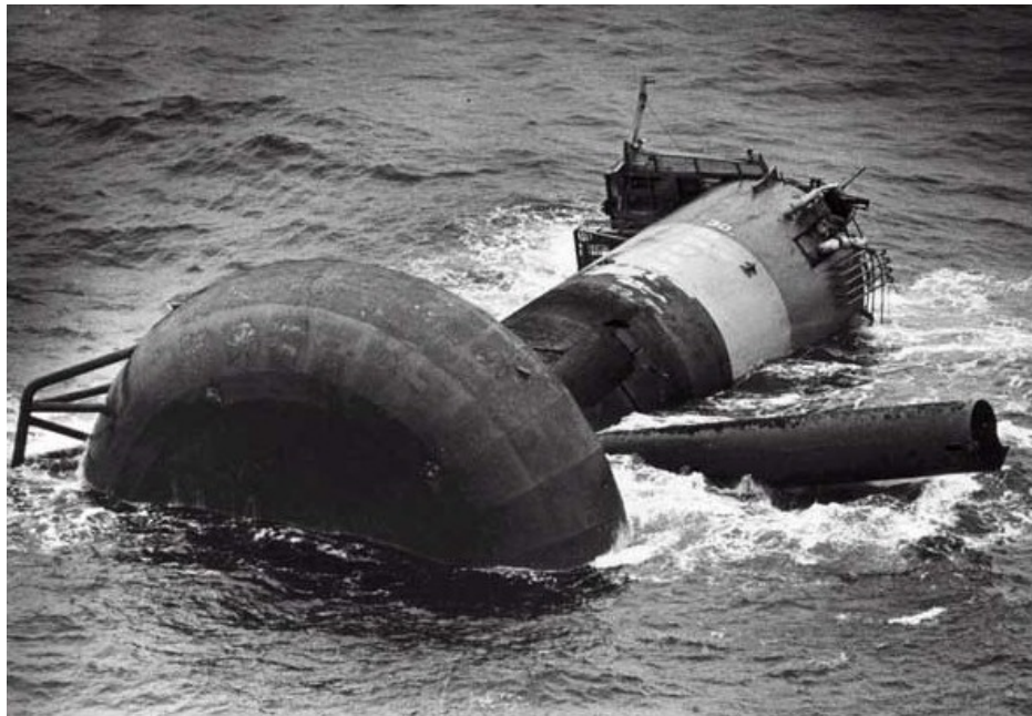
Figure 1.5 The collapsed leg floating above the sea surface after the accident
