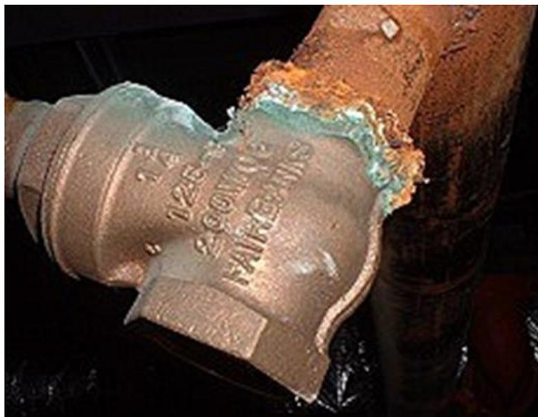
**Figure 3.12 Example of Galvanic Corrosion (InterNACHI, 2018)**
