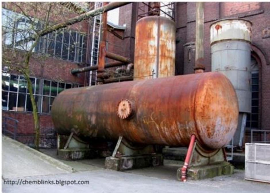
**Figure 3.3 Example of Uniform Corrosion (Chemblinks Blogspot, 2018)**
