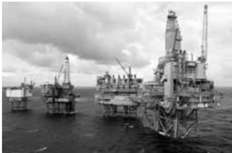
**Figure 2.7 Steel Platform Supporting Topside Facilities (Devold, 2013)**
