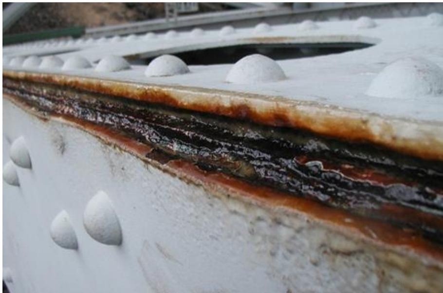
**Figure 3.7 Example of Crevice Corrosion (Steel Fabrication Services, 2018a)**
