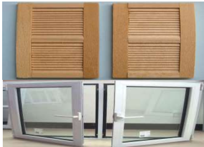
Figure 4. 24 Typical (a) Jalousie and (b) Aluminium panel/glazed window types in study area
