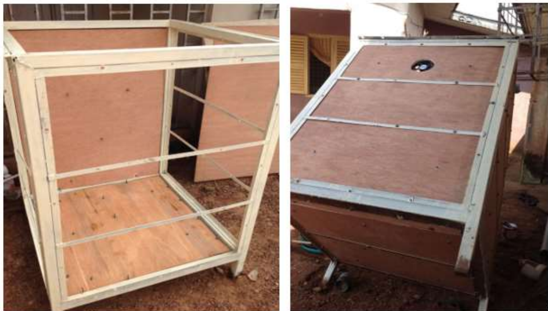
Figure 5. 12 Experimental Cell under Construction
