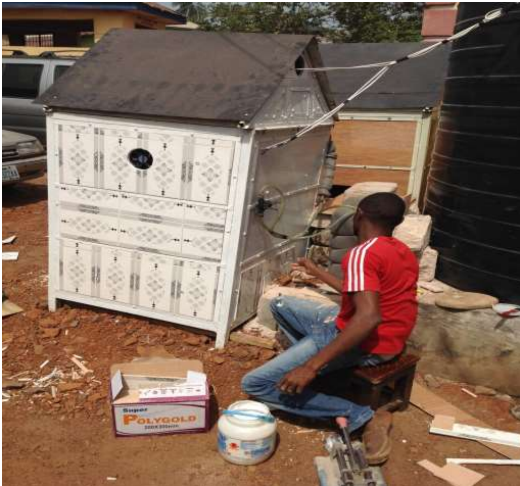
Figure 5. 16 External wall finishing on experimental cells PCS 1 and PCS 2
