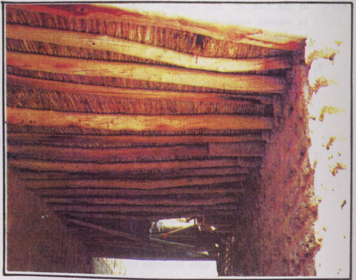
Fig. 56 : A photograph showing "al'chandel wood" trunks and "al'shererback" in a roof of a ground floor room (10).
