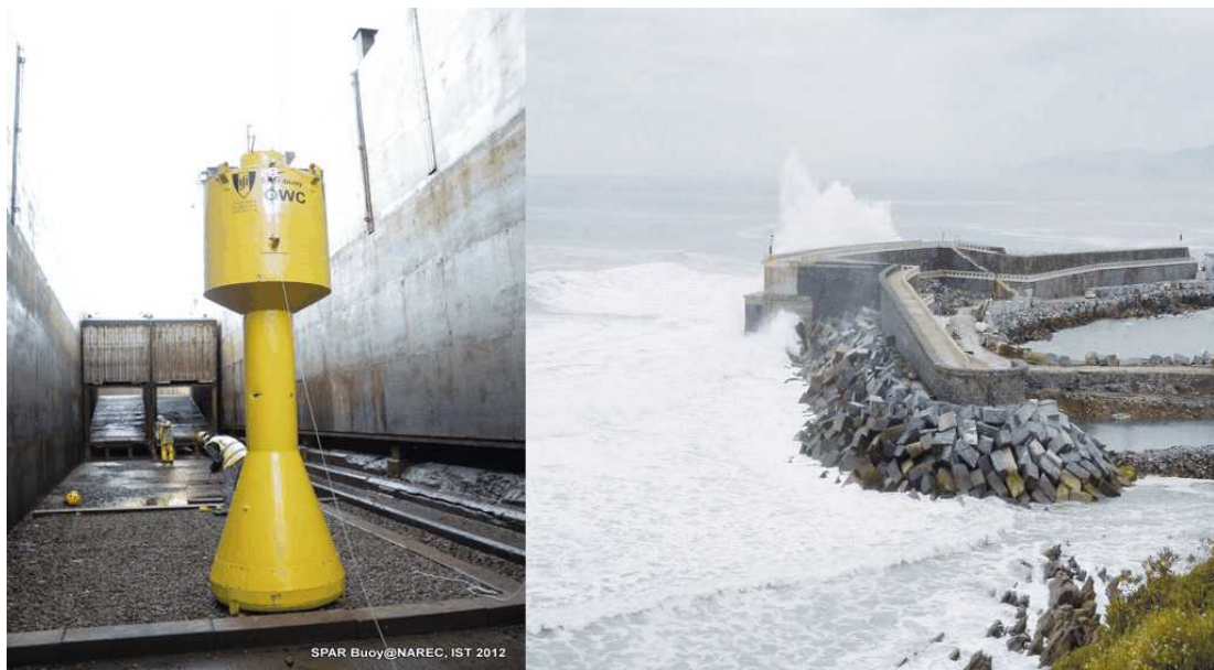
Figure 2.9: Sparbuoy OWC (left); Mutriku power plant during a storm (right). Figure is taken from TETHYS (2012)
