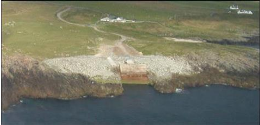
Figure 2.13: Wavegen LIMPET OWC plant. Figure is taken from Heath (2012).
