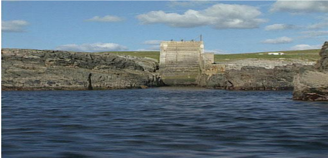
Figure 2.12: Queen's University Belfast 75kW demonstrator on Islay. Figure is taken from Heath (2012).
