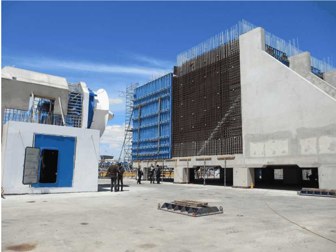
Figure 2.17: Reinforced concrete Greenwave device under construction
