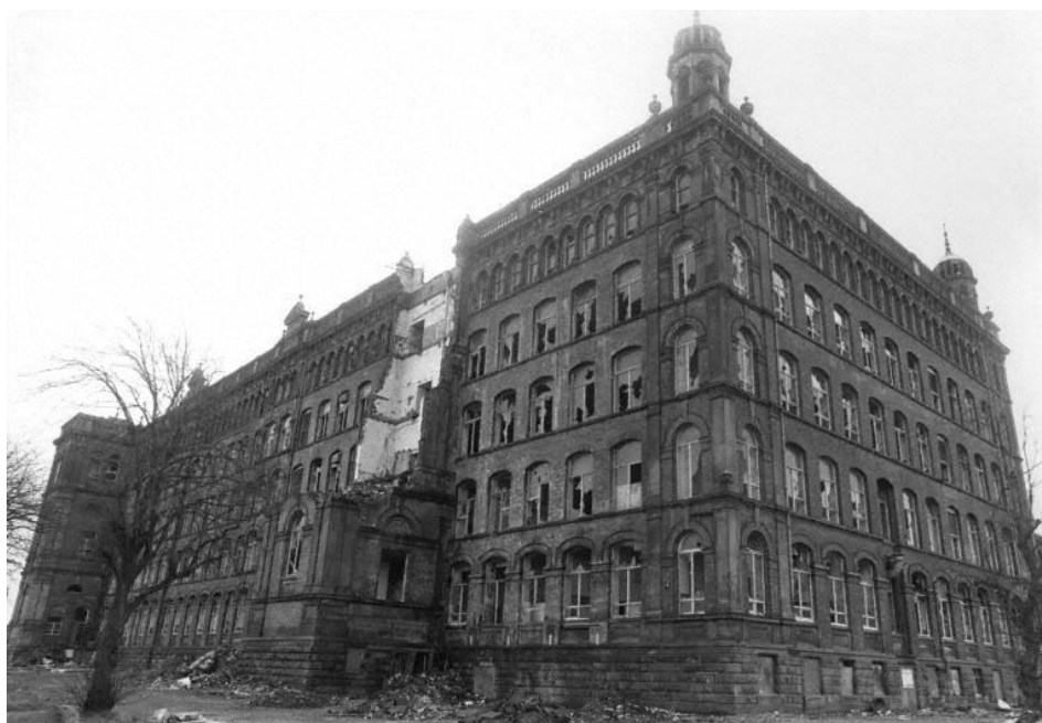
Figure 5.1: The derelict No.1 Spinning Mill, Ferguslie Mill.
