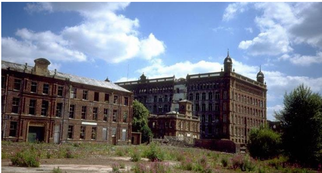
Figure 5.2: The derelict Ferguslie Mill.
