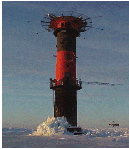
Figure 5.39: Norströmsgrund lighthouse (Bjerkas et al. (2009))
