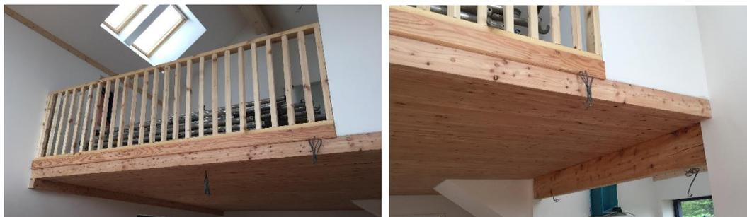
**Figure 9-5: Edge fixings around DLT panel.**
