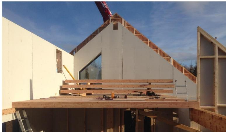
**Figure 9-2: Installation of panels.**
