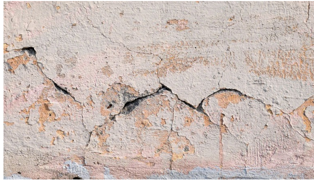
Figure 2.3: Concrete spalling adapted from [39]. The image dimensions are 780 \times 440 pixels, and the scale is set at 1cm : 20 pixels.
