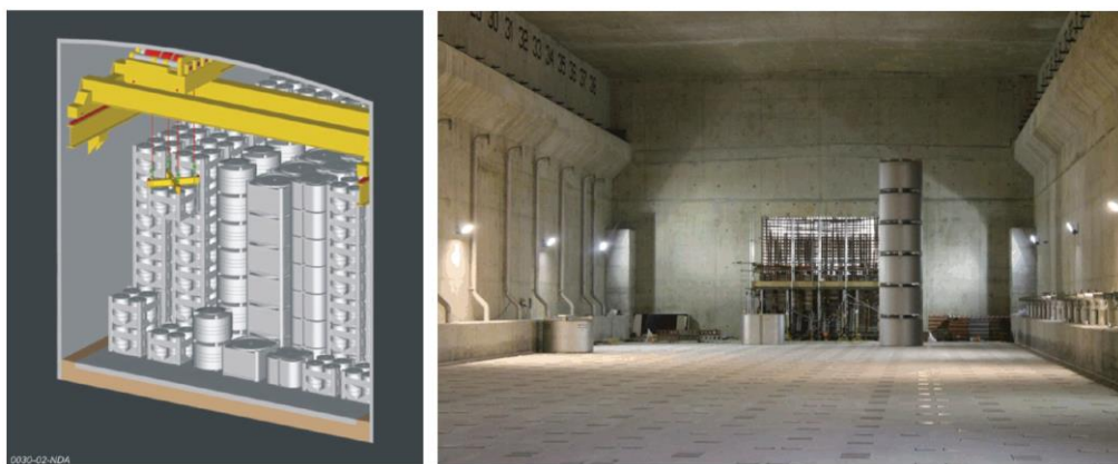
Figure 9: (Left) 3D visualisation of vault stacking [24]. (Right) Hunderson A ILW storage facility [27].
