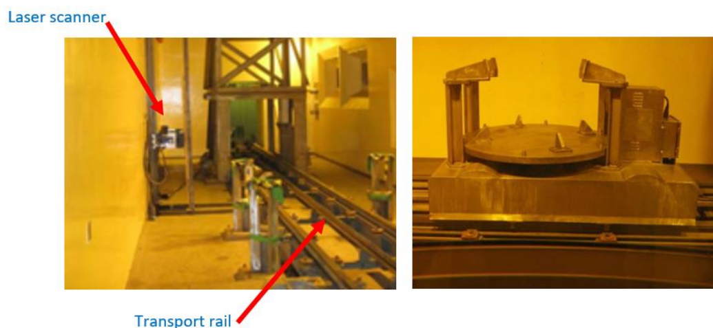
Figure 20: (Left) Geometrical laser scanner mounted in a wall inside EPS1, facing a transport rail on which the ILW are transported. (Right) The transport platform used to deliver the 500 L ILW drums to the laser scanner, the platform incorporated a turn table to rotate the drums and expose all their facets to the laser scanner field of vision [28].
