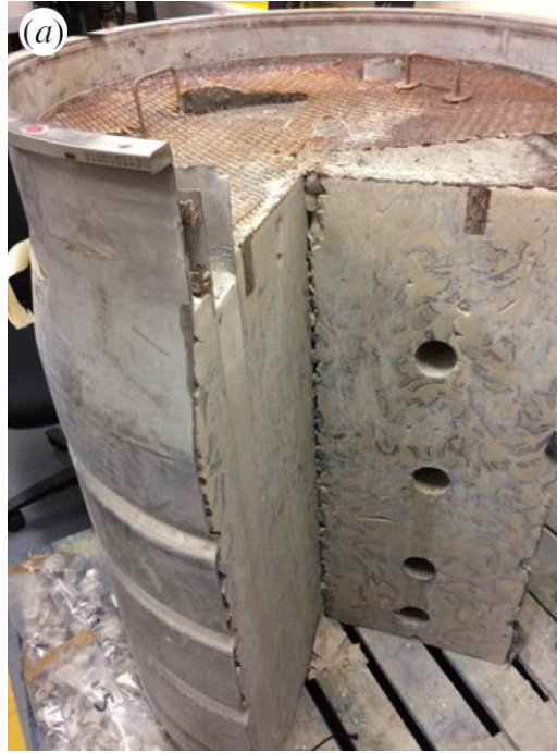
Figure 133: Showing potential gap between cement and the wall due to air bubbles [64].
