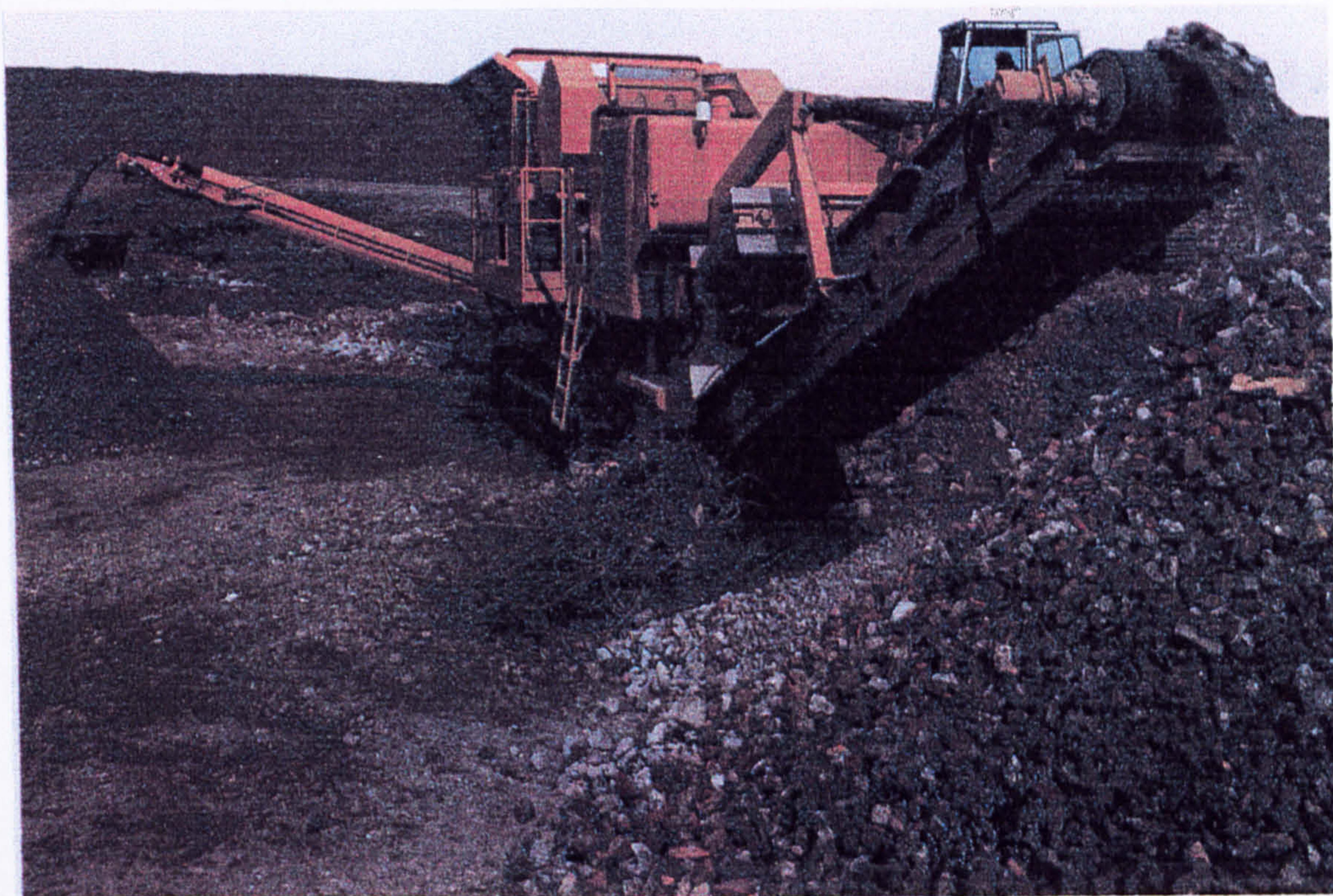
Fig. 3.1 Mobile plant for production of recycled aggregate.
