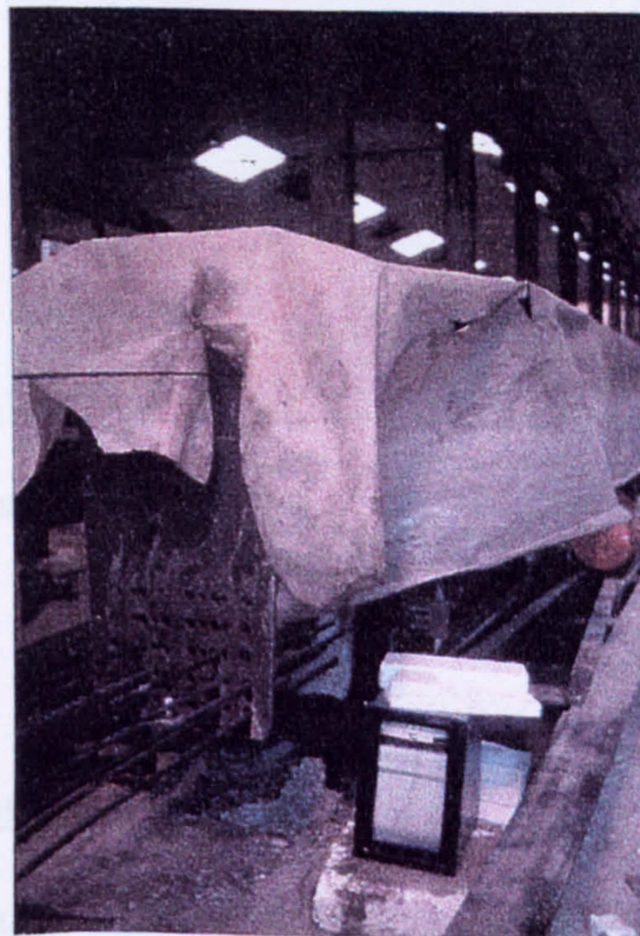
Fig. 5.5 Accelerating curing of the pre-stressed beams.
