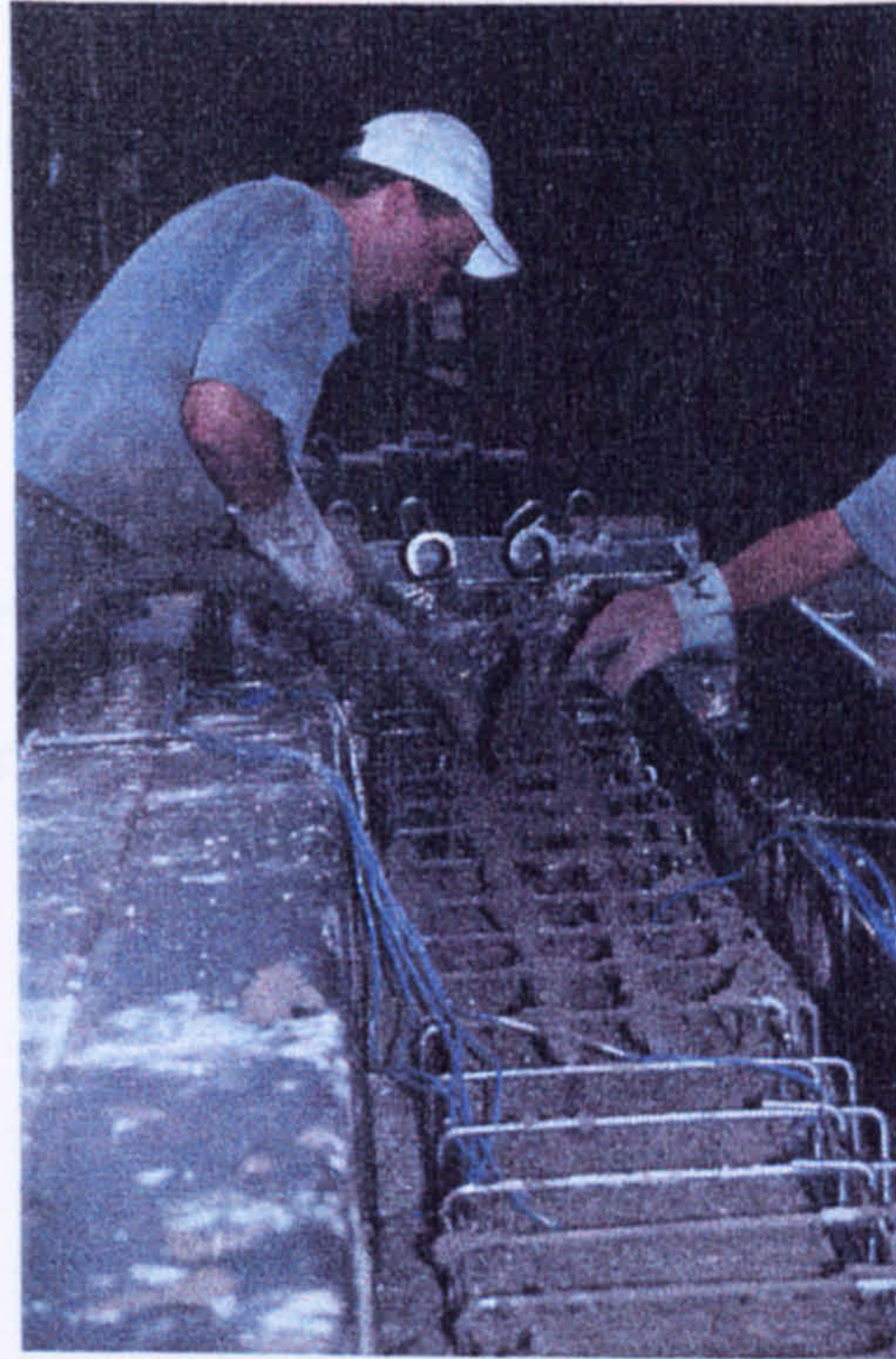
Fig. 5.4 Casting and vibration phases.
