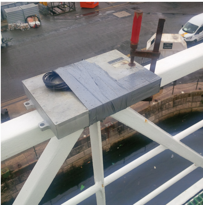
(b) View on logger position from walkway
