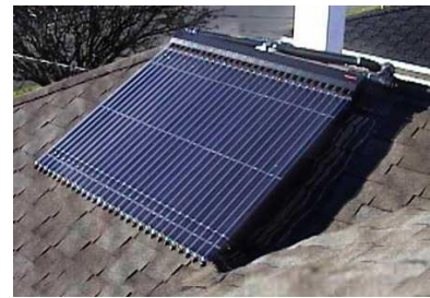
Figure 6 - Evacuated Tube Collector (59)
