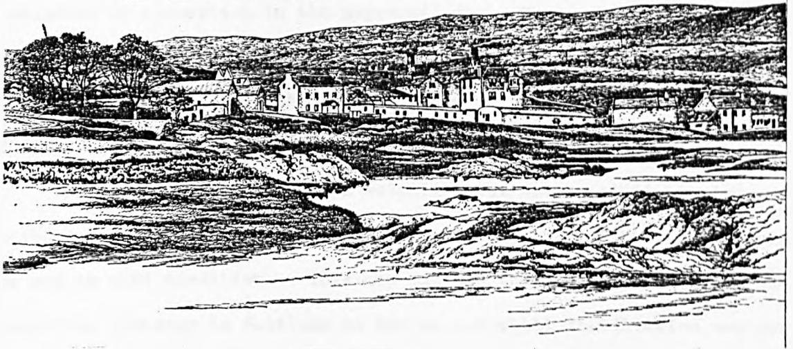
Jura distillery, c. 1886. James Ferguson & Sons. Erected by the laird, Campbell of Jura, and tenanted by several entrepreneurs, it was dismantled c. 1910-20, and has been reconstructed.
