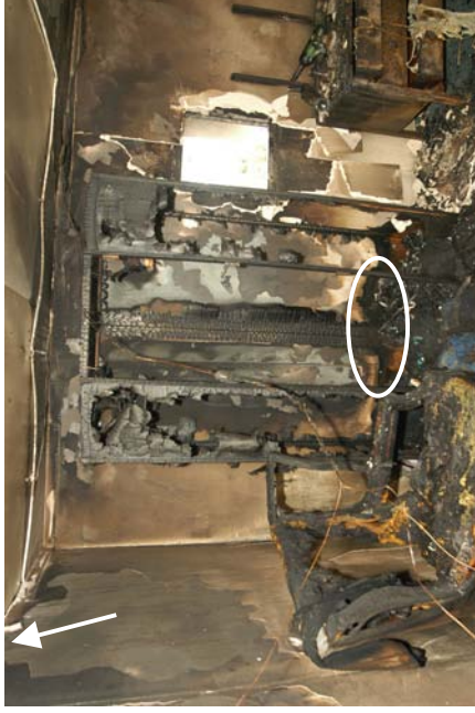
Figure 64 - Post-fire photograph detailing the damage to the wardrobe. The white arrow is the location of exhibit 005.
