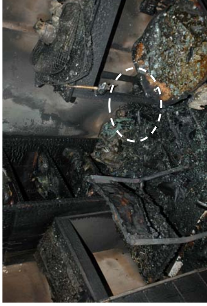
Figure 66 - Post-fire view of the area of origin for this fire [147].
