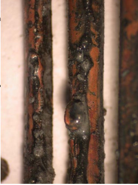
Figure 964 - Microscope image of exhibit 140. The arcing damage has affected the live and smaller earth conductor. The damage extends to 7mm in length and is a good example of arcing through char.
