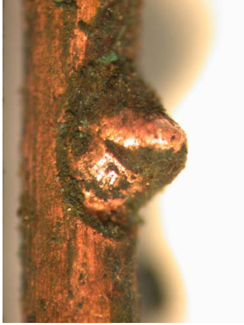
Figure 641 - 40x magnification of the notch with a bead within detailing the clear demarcation between the arcing damage and the undamaged conductor.
