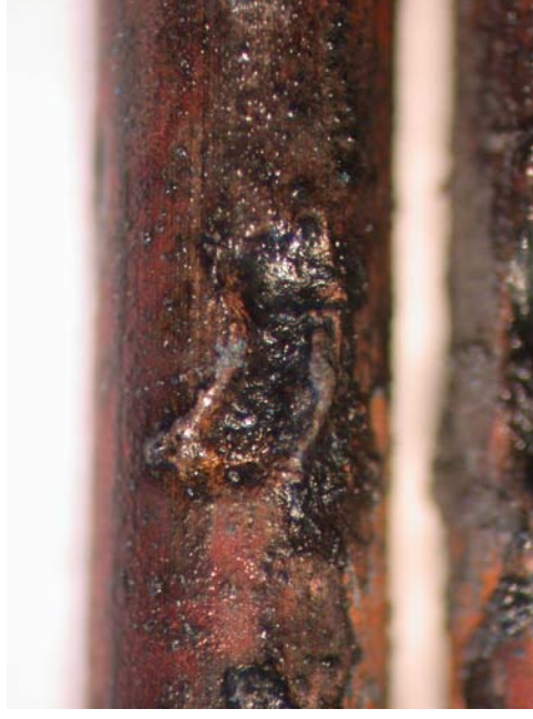
Figure 277 - View of the notch damage to the 2.5mm 2 conductor at 40x magnification.
