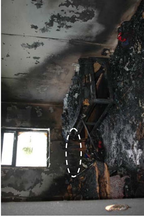
Figure 834 – Post-fire view of the experiment. There are burn patterns on the rear and right wall of the compartment.
