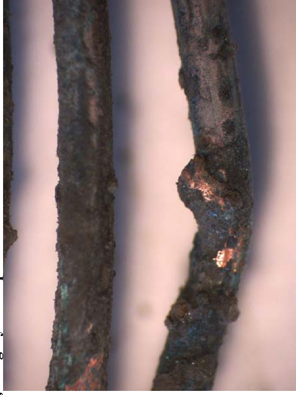
Figure 282 – Microscope image at 20x magnification detailing the arcing damage to the bottom conductor in figure 281.
