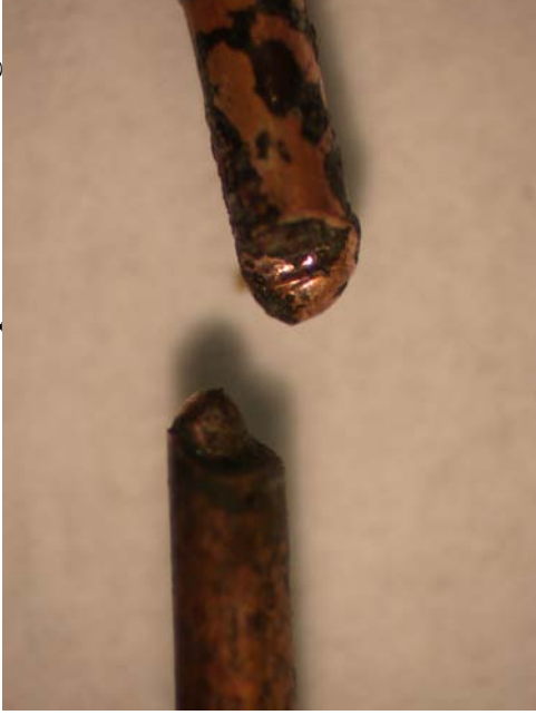
Figure 466 - Microscope image of exhibit 067 detailing the two severed ends of the one conductor with metallic damage.
