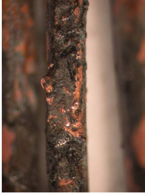
Figure 607 - Microscope image of the second conductor with arcing category A.
