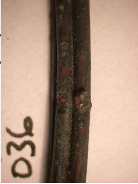
Figure 248 - Microscope image of exhibit 036. The localised metallic damage involved two conductors. One with a notch and the other with a bead within a notch.
