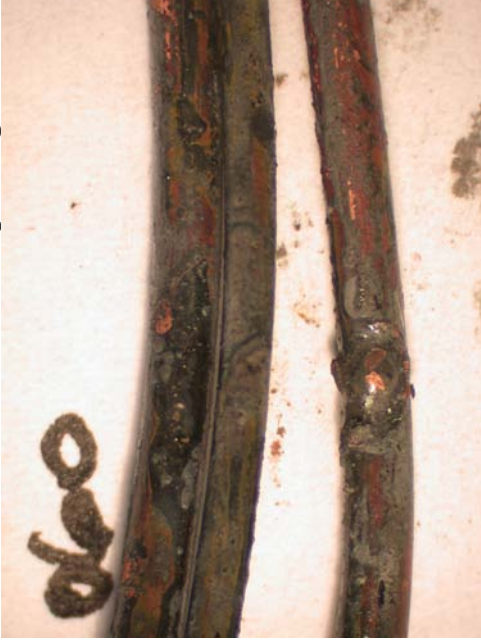
Figure 409 - Microscope image of exhibit 060. The arcing damage affects one of the three conductors with a bead within a notch.
