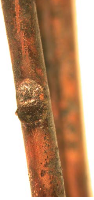
Figure 763 - 20x magnification of the smaller notch. There is a demarcation area at the edge of the notch between the arcing damage and the undamaged conductor.
