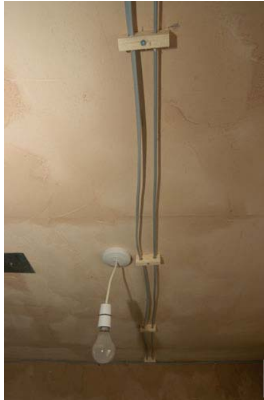
Figure 45 –Timber blocks simulating floor joists used to support the cables.
