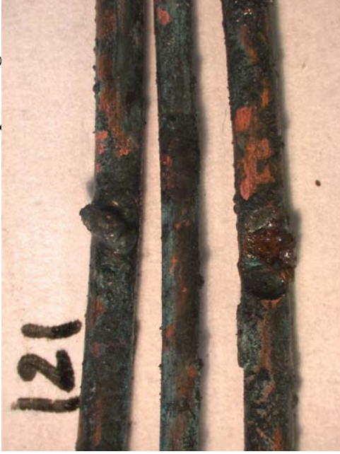
Figure 807 - Microscope image of exhibit 121. The two 2.5mm 2 conductors (live & neutral) each have a notch with a bead within the notch. The top conductor's bead is protruding up from the surface.
