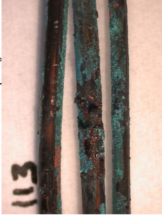
Figure 753 - Microscope image of exhibit 113. The arcing damage affected one conductor with a notch and copper splatter around the notch edge.
