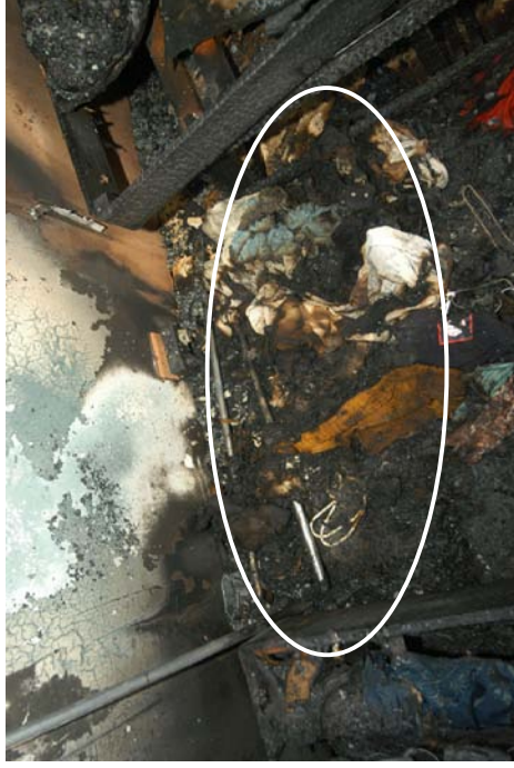
Figure 508 - Close-up photograph of the fire's area of origin. The fire was ignited with a flame to simulate a faulty fan heater below portable clothes rail full of clothing.
