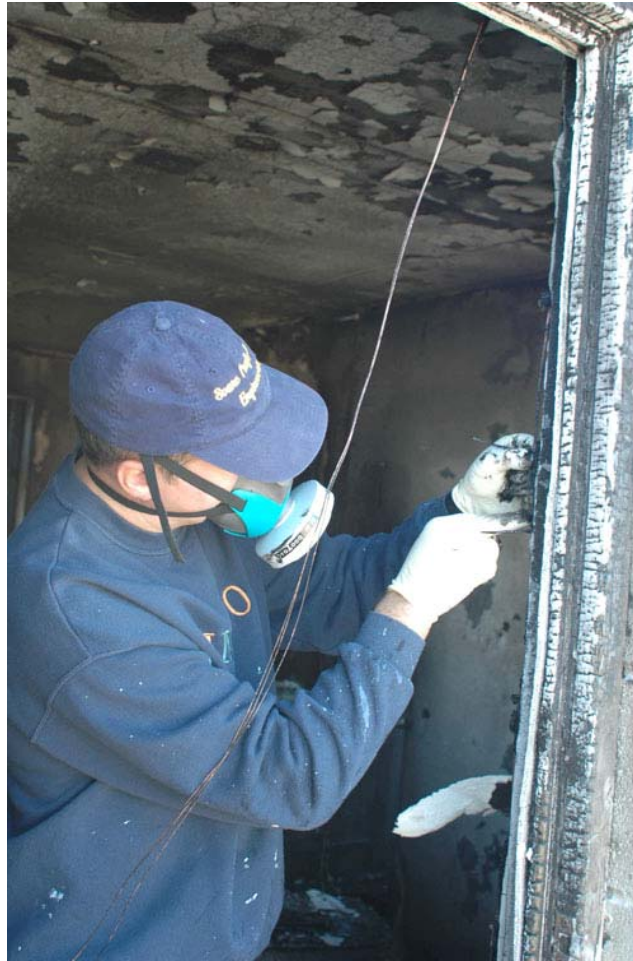
Figure 57 – Examination of the copper conductors post-compartment fire [146].
