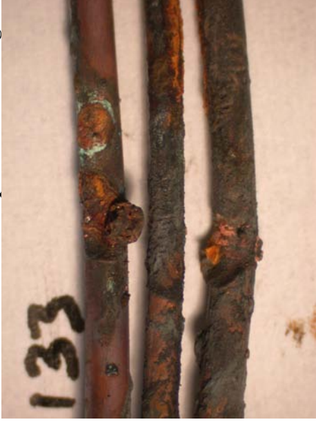
Figure 905 - Microscope image of exhibit 133. The two 2.5mm 2 conductors (L&N) had arcing damage. The conductors had arced across the fixing screw.
