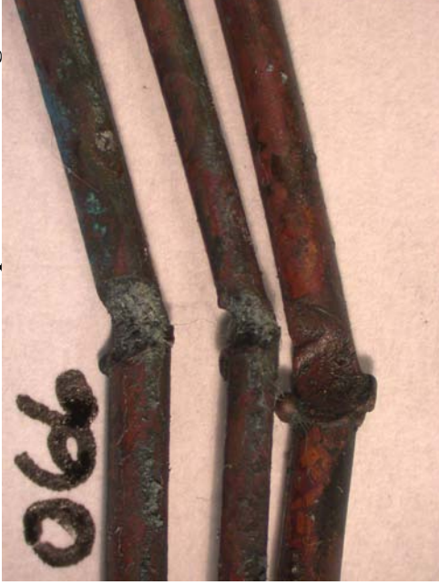
Figure 462 - Microscope image of exhibit 066 with notch damage to all three conductors.
