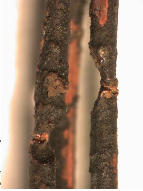
Figure 236 – 20x magnification of the top and bottom conductors detailed in figure 235. Note the cracks in the metal surface below the notches.
