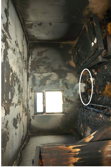
Figure 507 - Post-fire photograph detailing the fire's area of origin located adjacent to the rear wall and between the beds.
