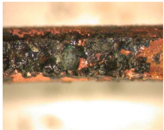
Figure 36 – A close-up of a section of figure 35 showing the arcing through carbonised cable insulation in more detail.
