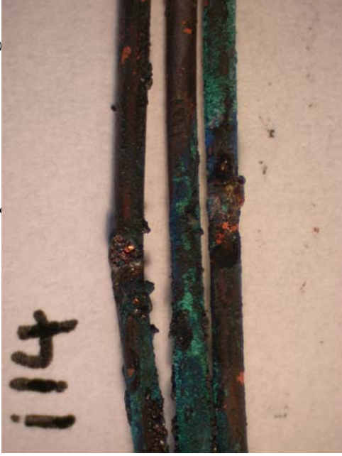
Figure 755 - Microscope image of exhibit 114. The arcing damage affected two of the three conductors. Each conductor has a notch with a bead at the edge.
