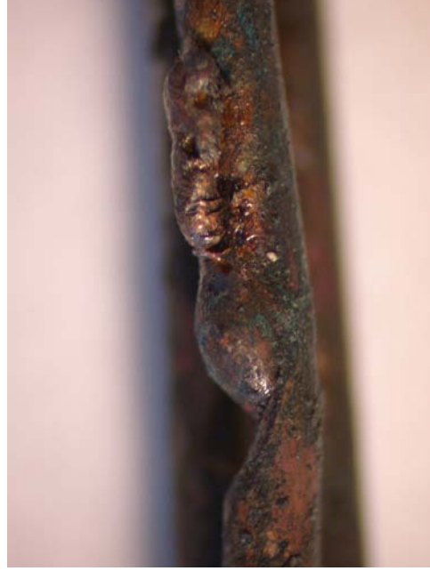
Figure 592 – The exhibit has been rotated 180 degrees detailing the opposite side of the arcing damage to figure 591.
