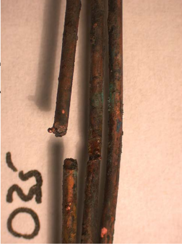
Figure 238 - Microscope image of exhibit 035. The metallic damage has affected two conductors. The top conductor is severed and the bottom conductor has a notch.
