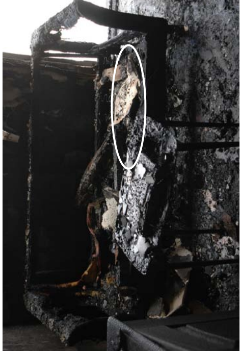
Figure 772 - Post-fire view of the three-seat settee next to the entrance door that was the dominant fire plume in the early development of this fire.
