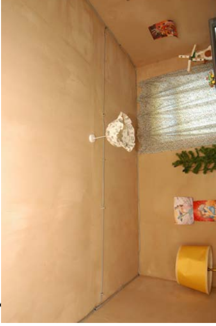
Figure 647 - Pre-fire photograph of the ceiling area detailing the wiring located above the fire's area of origin.
