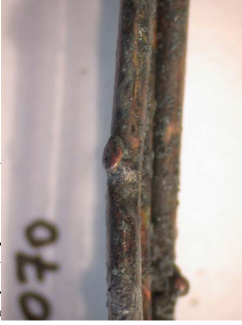
Figure 490 - Image of the two conductors with arcing damage. Depth of field issues renders one conductor out of focus in this image.
