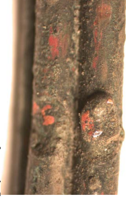
Figure 249 – Microscope image at 20x magnification detailing the damage to the two conductors.
