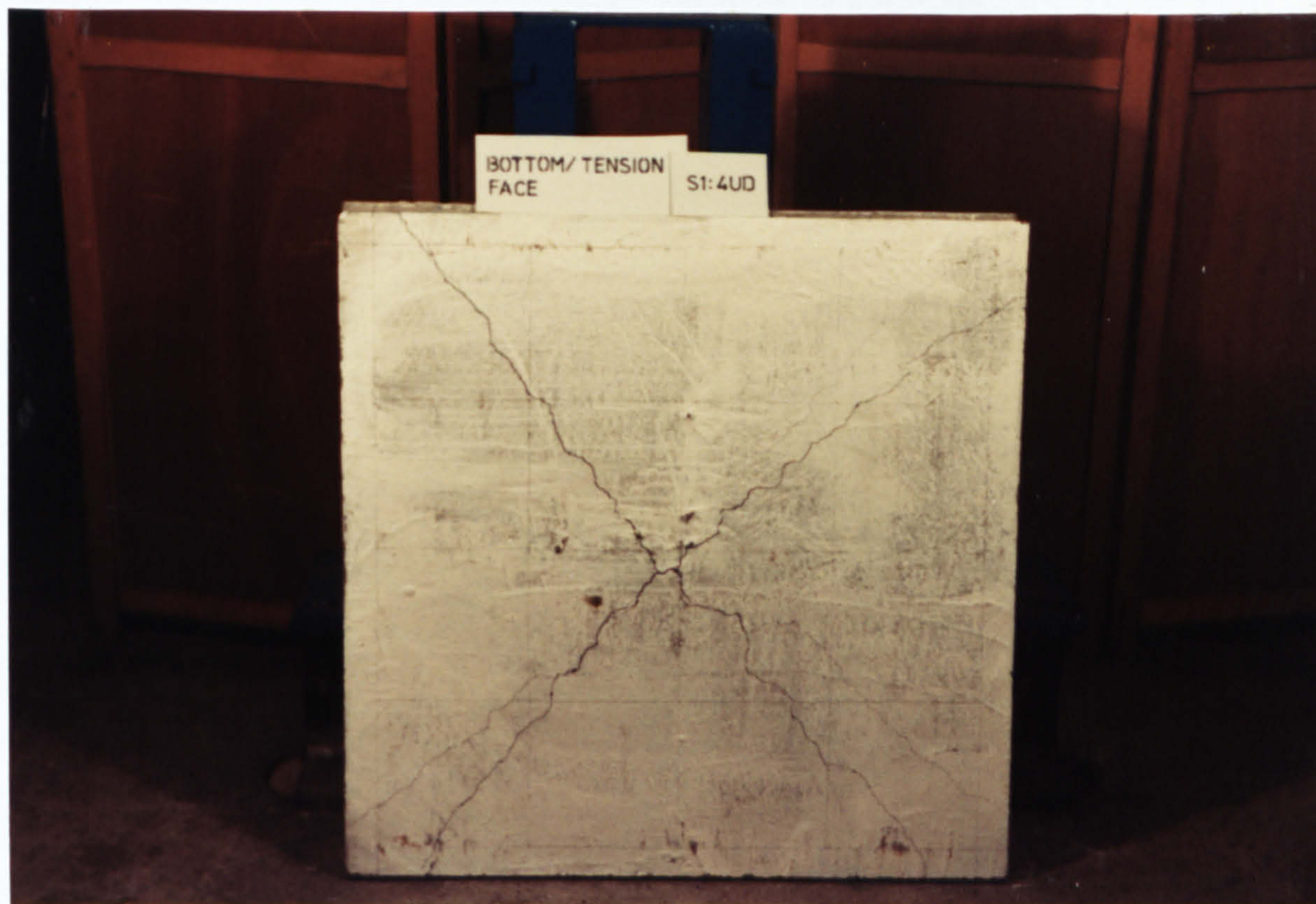
Plate 6.7 Crack Patterns at Failure on the Tension Face of Model S14UD.
