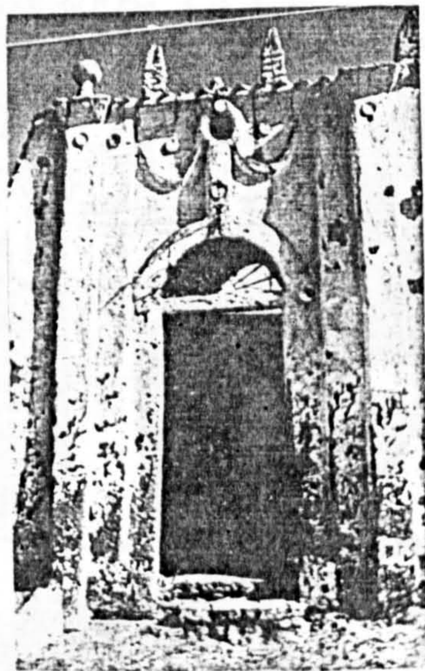
(Plate 3) "View of Nubian Women's Entrances". In "Hassan Fathy", ed. Richards, J. Architecture Press, London (1985).
