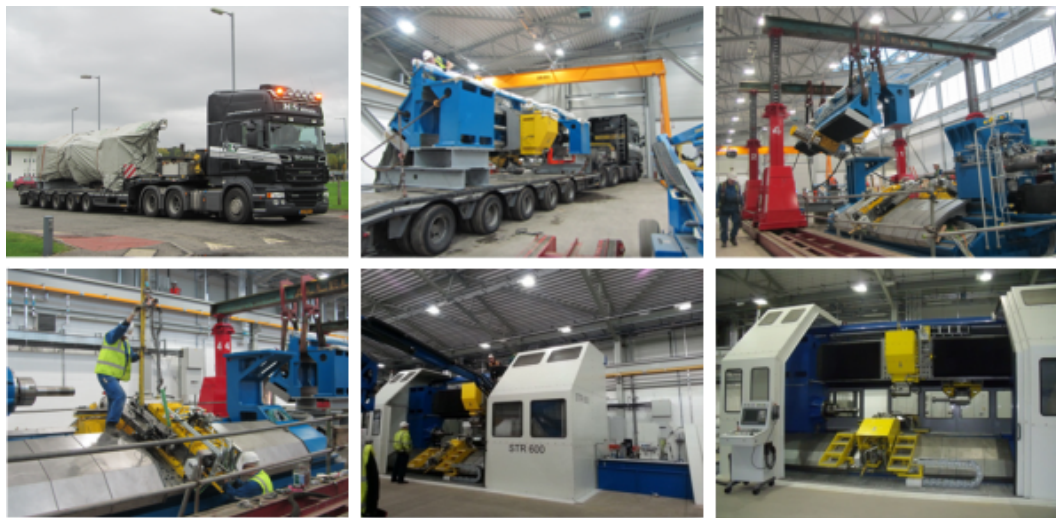
Figure C.1: Delivery and installation of the flow former at the AFRC.
