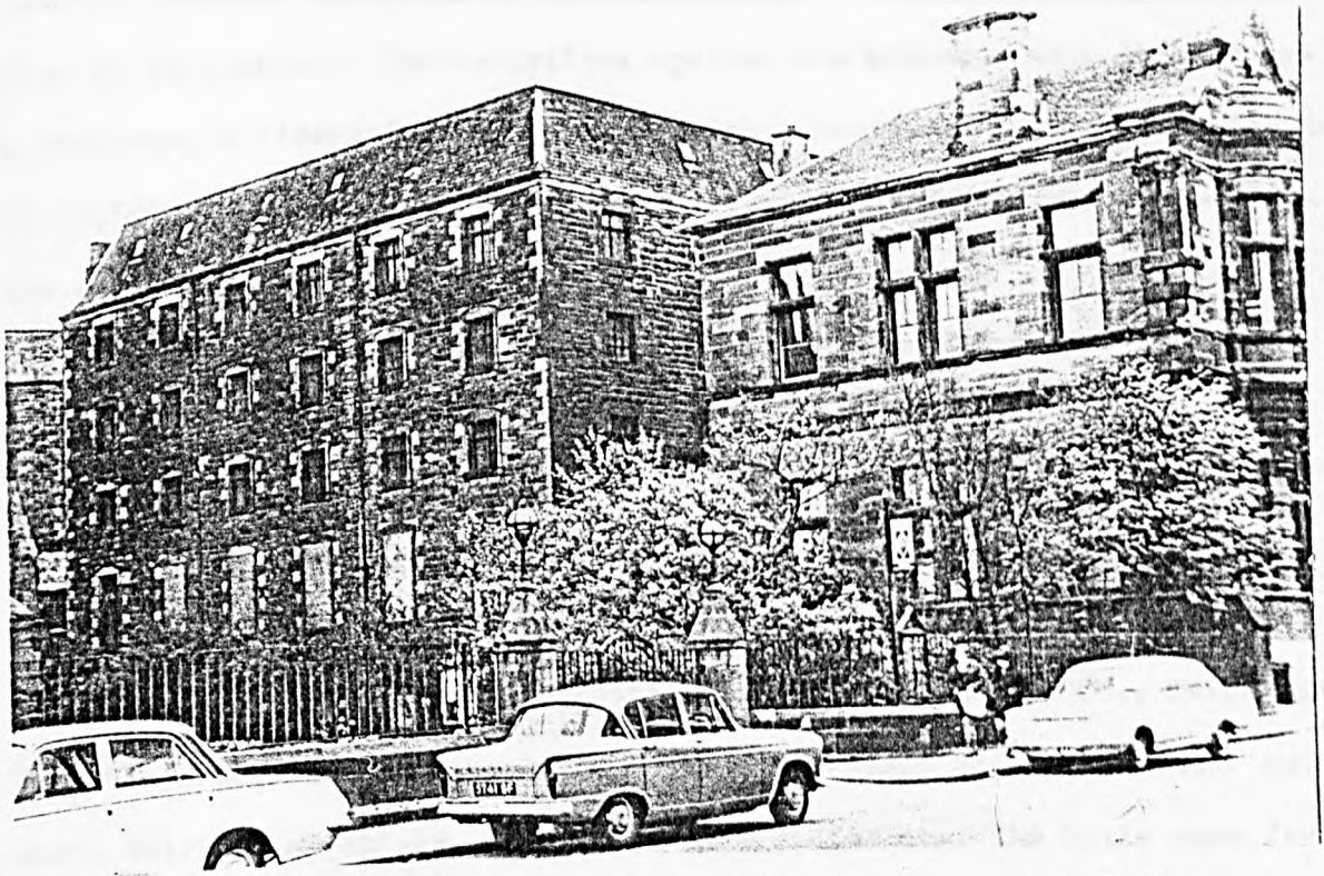
The imposing warehouses behind the former offices of Pattisons Ltd. (From A.E. Glen, B.Sc.)
