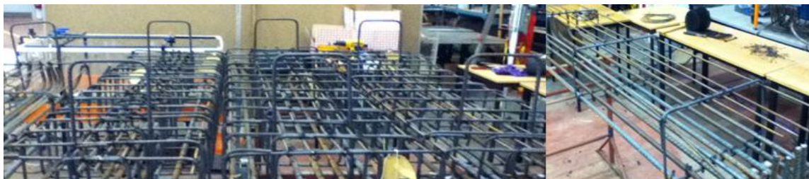
Figure 7.4: Typical Steel Cages for the Beams in Test-Series "1".
