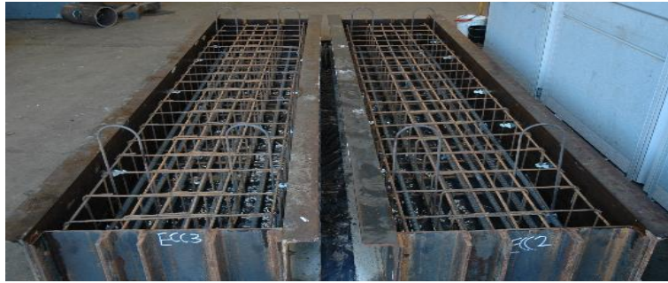
Figure 5.5: Steel Shutters used for the Beam Specimens in Test-Series "A".
