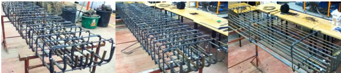
Figure 9.4: Typical Steel Cages for the Beams in Test-Series "2".
