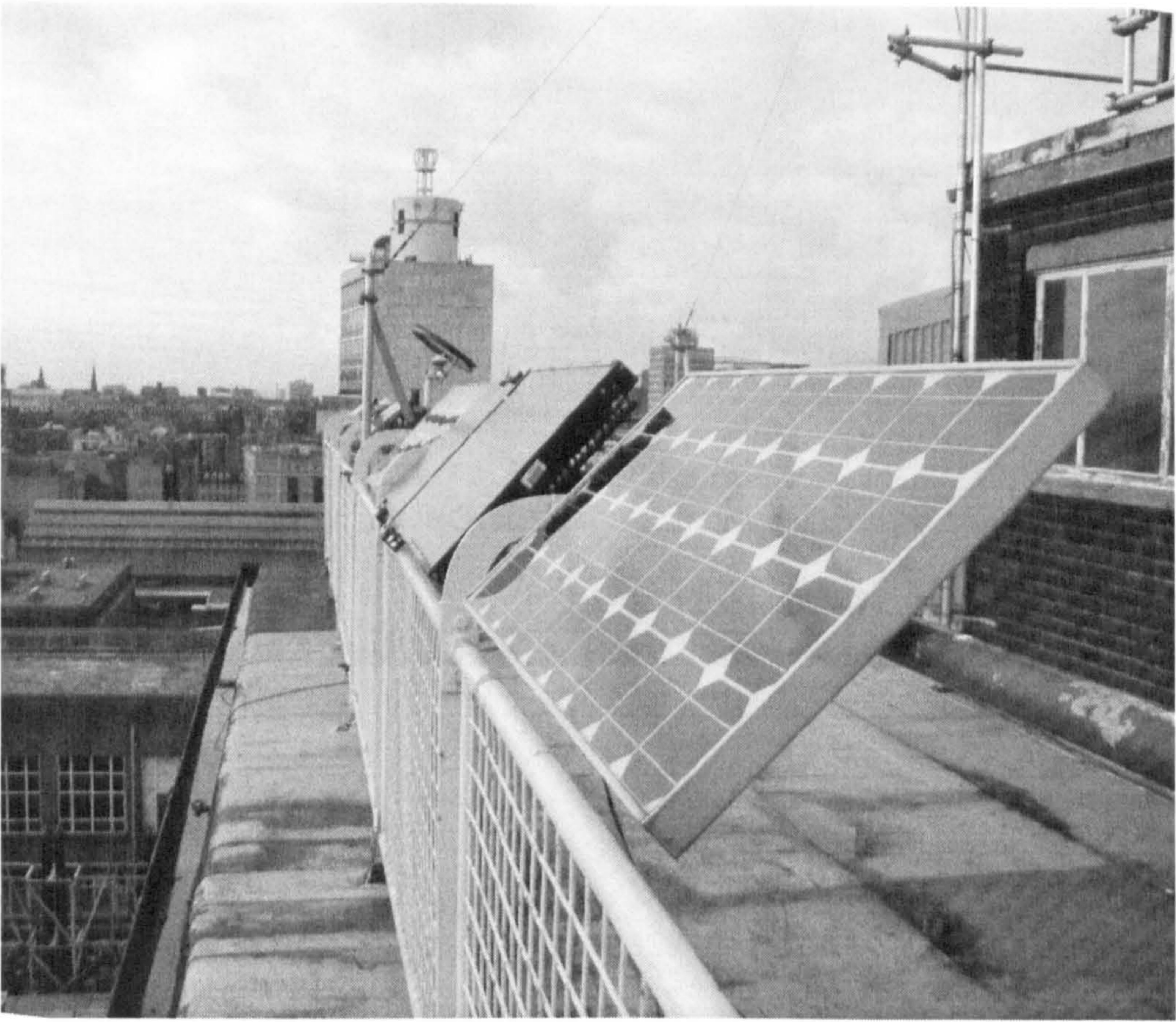
(Fig. 6.3: PV Modules mounted on roof)
