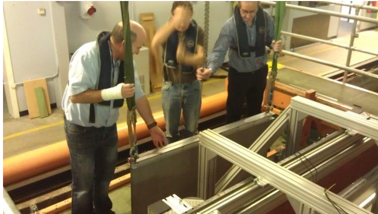
Figure 4.12: Installation of the Reference Plate.
