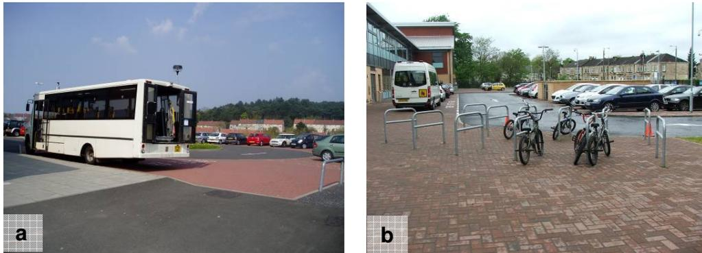
Image 4.67: Examples of (a) tarmac paving with white contrasting path (b) red monoblock paving.
