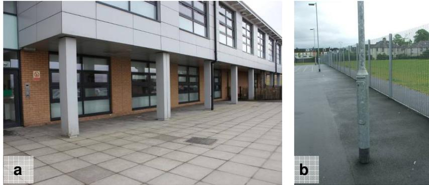
Image 4.66: Examples of (a) columns and (b) posts which are not marked with colour contrasting bands.
