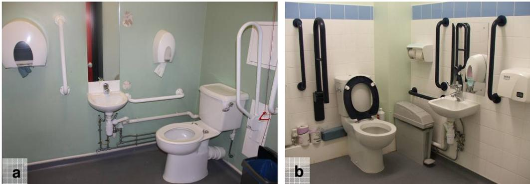
Image 4.56: Accessible WCs showing (a) grab rail broken from wall and no colour contrasting fittings & (b) colour contrasting fittings.
