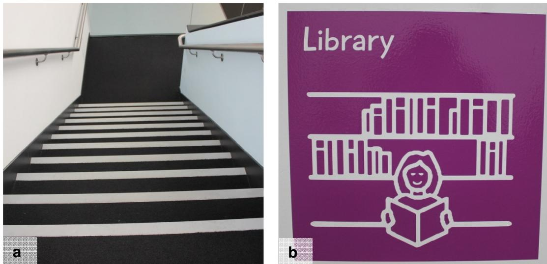
Image 6.25: (a) Stairs with colour contrasting stair nosings & (b) signage with dark background, large colour contrasting sans-serif typeface & symbol adapted from Boardmaker.
