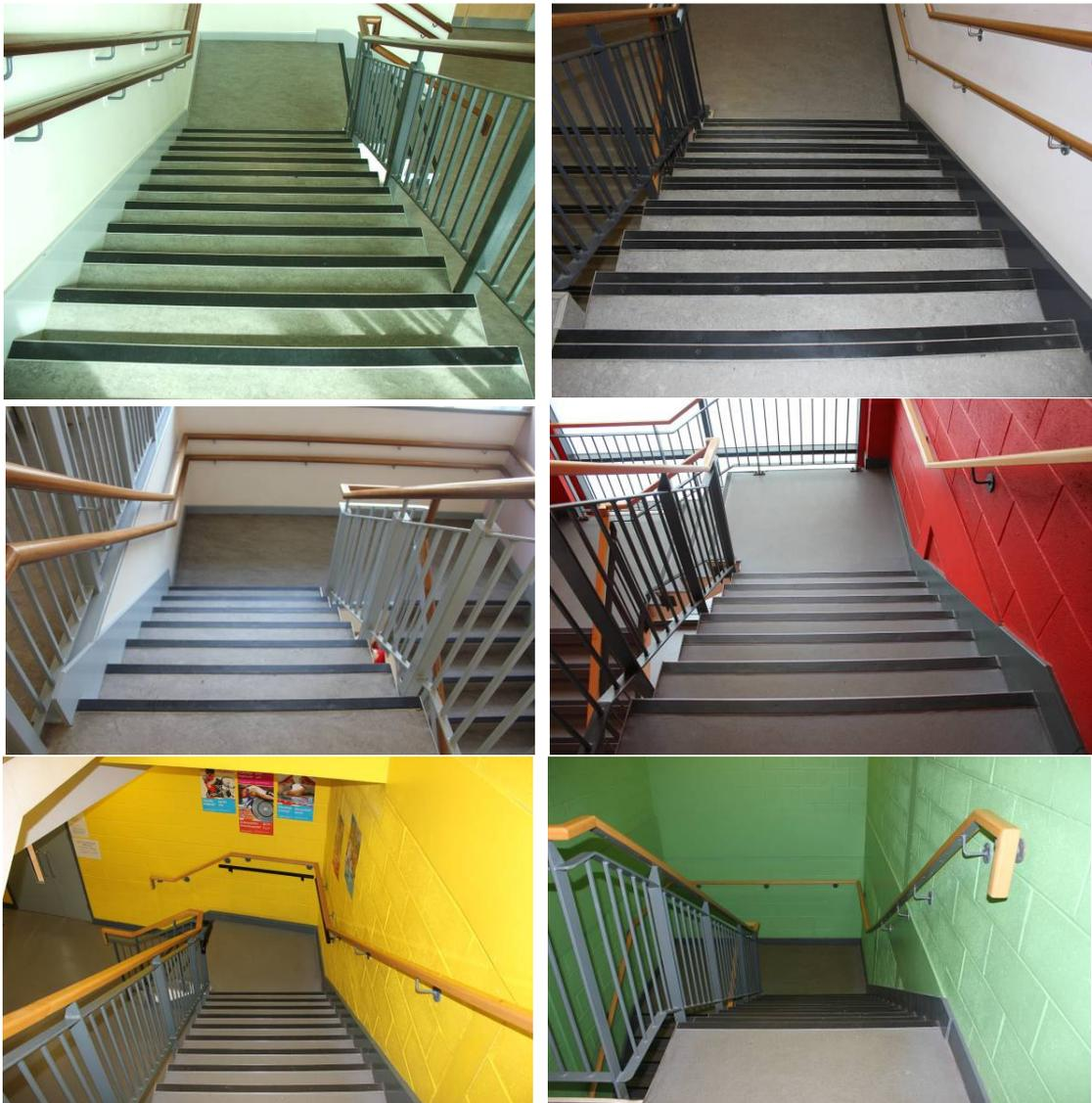
Image 4.24: Various colour combinations for floor finish, stair nosing, wall and handrail
