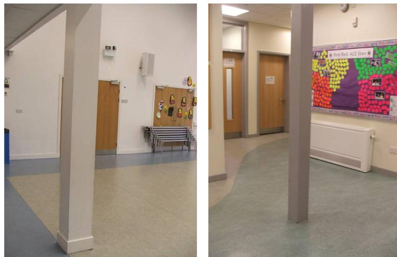
Image 4.17: Examples of columns which blend in with the background
