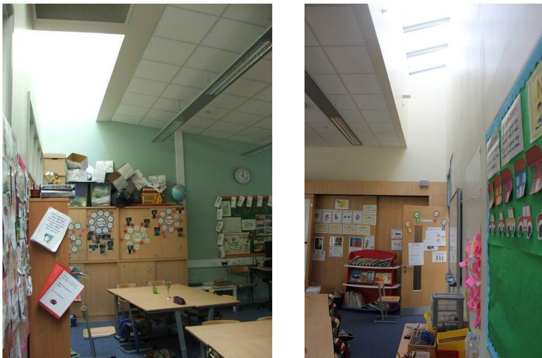
Image 4.33: Photos showing skylight along interior wall of upper floor classrooms.
