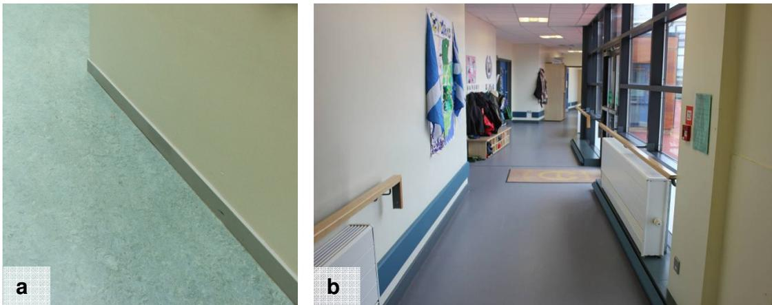
Image 4.18: Example of (a) light coloured floor which does not contrast well with the grey skirting board & (b) good contrast between wall and floor, but not between skirting board and floor.
