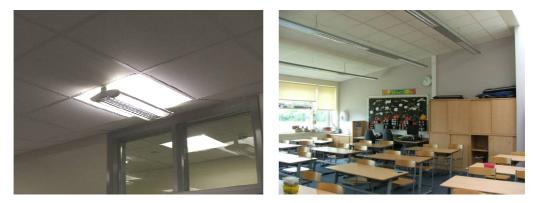
Image 4.37: Pirie Park Primary, examples of light fittings which project light both upwards and downwards.
