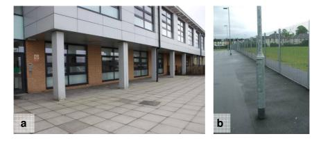
Image 4.66: Examples of (a) columns and (b) posts which are not marked with colour contrasting bands.
