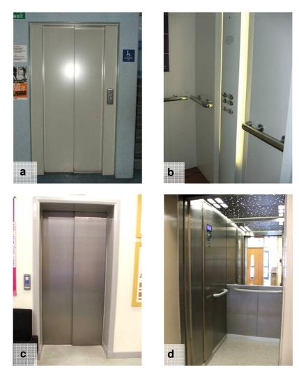
Image 4.23: (a) and (b) typical lift doors demonstrating the lack of contrast between door and wall surface, (c) lift control panel in refurbished school and (d) typical lift interior in new schools with shiny reflective surface and buttons which do not contrast.
