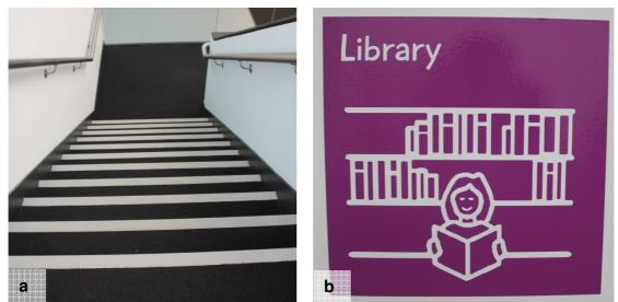
Image 6.25: (a) Stairs with colour contrasting stair nosings & (b) signage with dark background, large colour contrasting sans-serif typeface & symbol adapted from Boardmaker.
