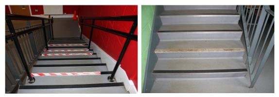
Image 4.29: Examples of poor quality construction with stair nosings coming off stairs at two schools.
