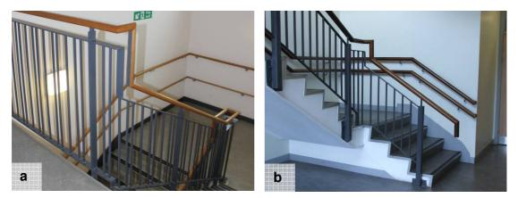
Image 4.26: Changes in height of handrail at (a) the landing and beginning of stair (b) other junctions throughout the stairway.
