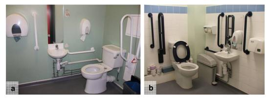
Image 4.56: Accessible WCs showing (a) grab rail broken from wall and no colour contrasting fittings & (b) colour contrasting fittings.
