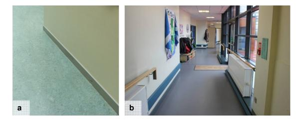
Image 4.18: Example of (a) light coloured floor which does not contrast well with the grey skirting board & (b) good contrast between wall and floor, but not between skirting board and floor.
