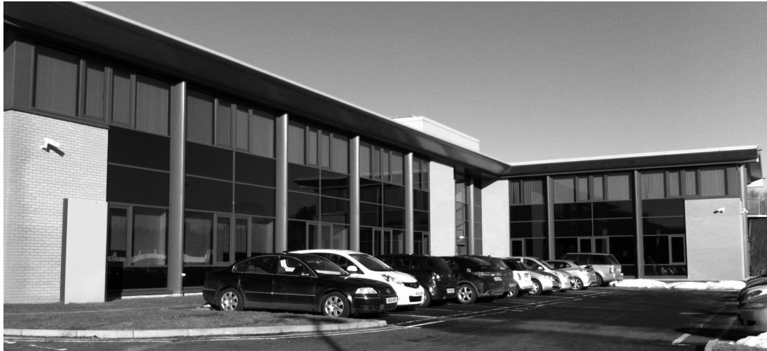
Figure 4.1 The Case Study Building.
