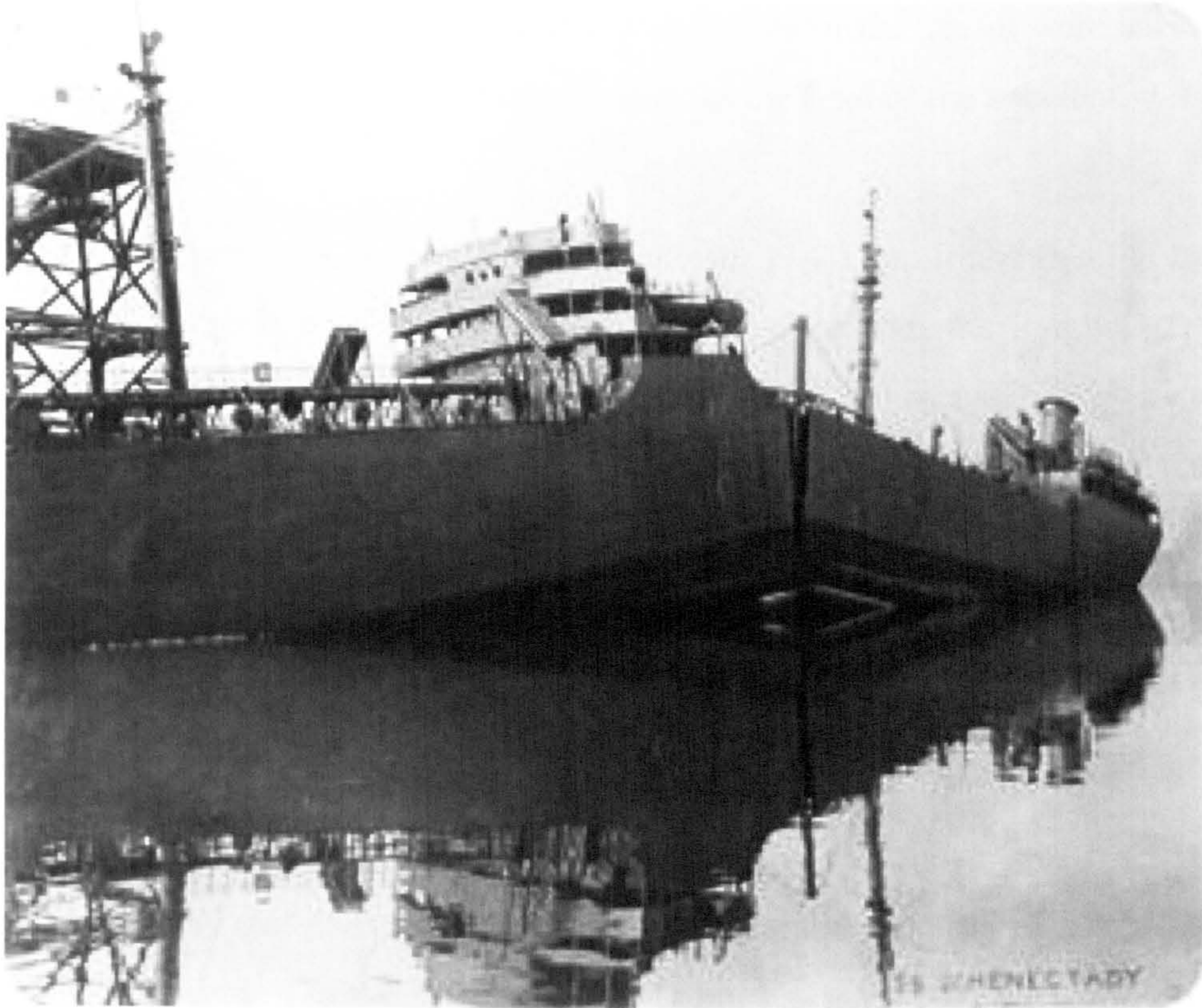
Figure 1-2 Example of Liberty ship suffering brittle fracture whilst in dock
