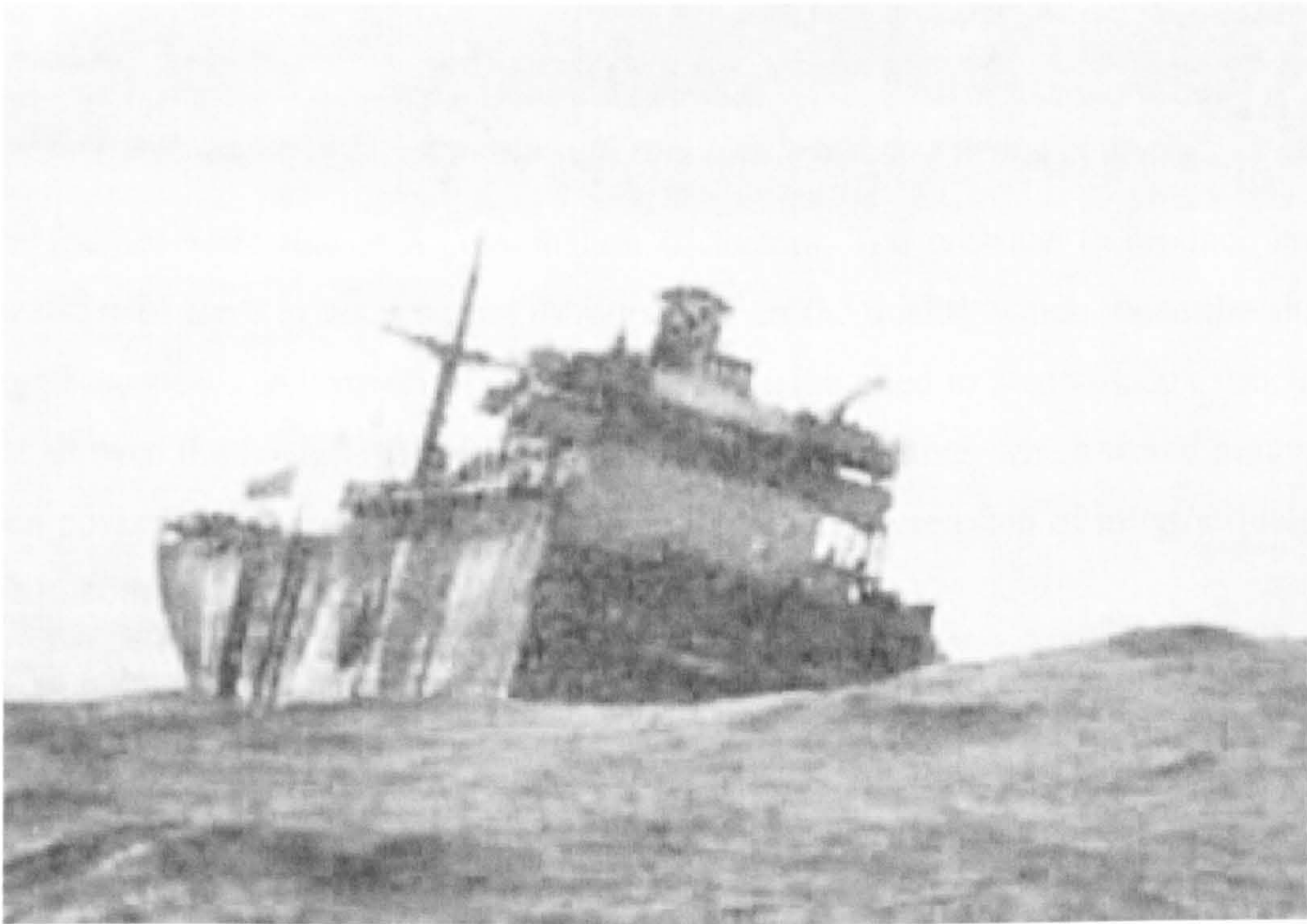
Figure 1-1 Brittle fracture of Liberty ship whilst at sea
