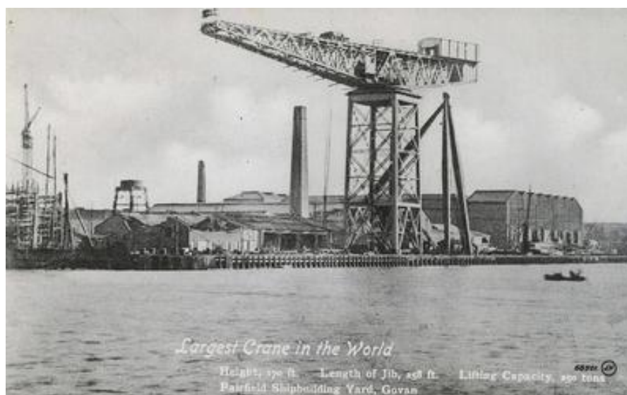
Figure 9 - Postcard featuring the Fairfield Crane, c1911, next to the now outdated and soon to be removed shear-legs system close by. ©Glasgow Museums
