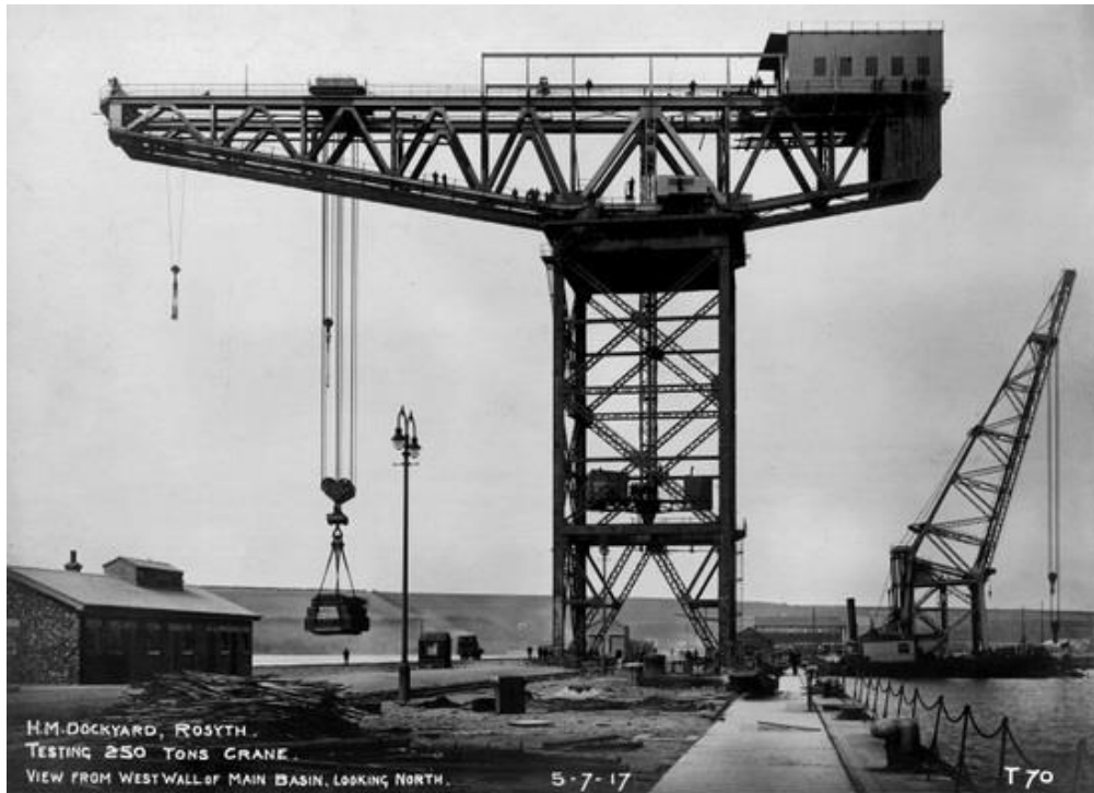
Figure 2 - The newly built 250 ton giant cantilever crane in Rosyth, whilst being tested. 05/07/1917. ©Historic
