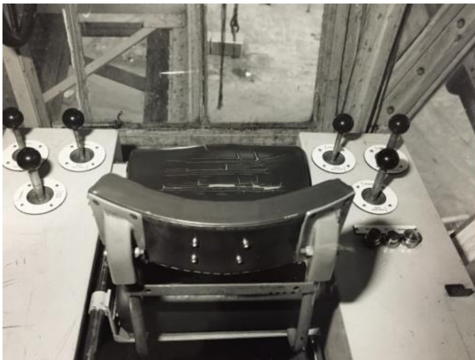
Figure 10 - The operator's seat and controls, Fairfield crane, 1990. ©Historic Environment Scotland
