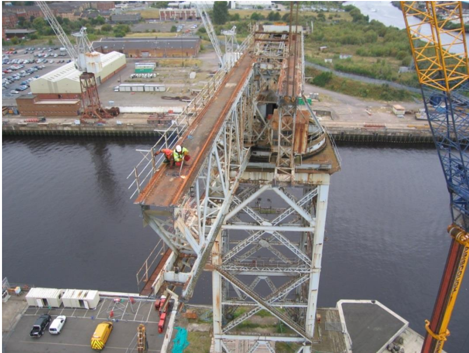
Figure 16 – Construction workers dismantling the Fairfield crane, 27 th October 2007.
