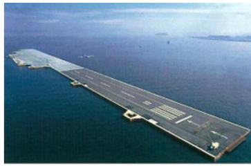
(a) Mega floater in Tokyo Bay
