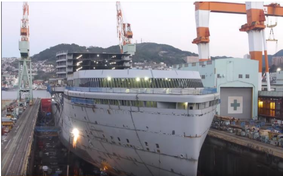
Figure 2-6 Block erection in dry dock
