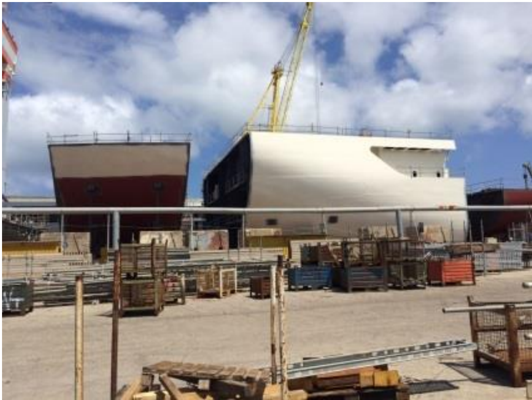
Figure 2-4 Grand blocks at a shipyard (Passenger ship)
