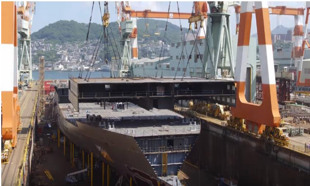
Figure 2-1 Block weight depends on the crane capacity available
