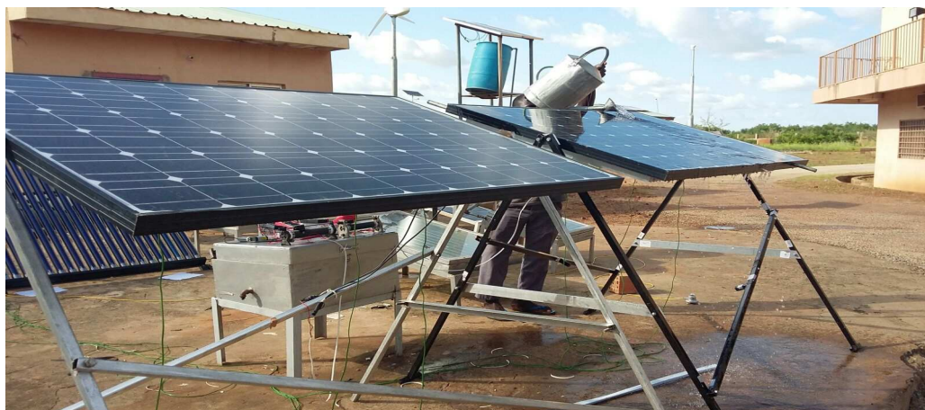
Figure 4-7 Manual water spraying of the module.
