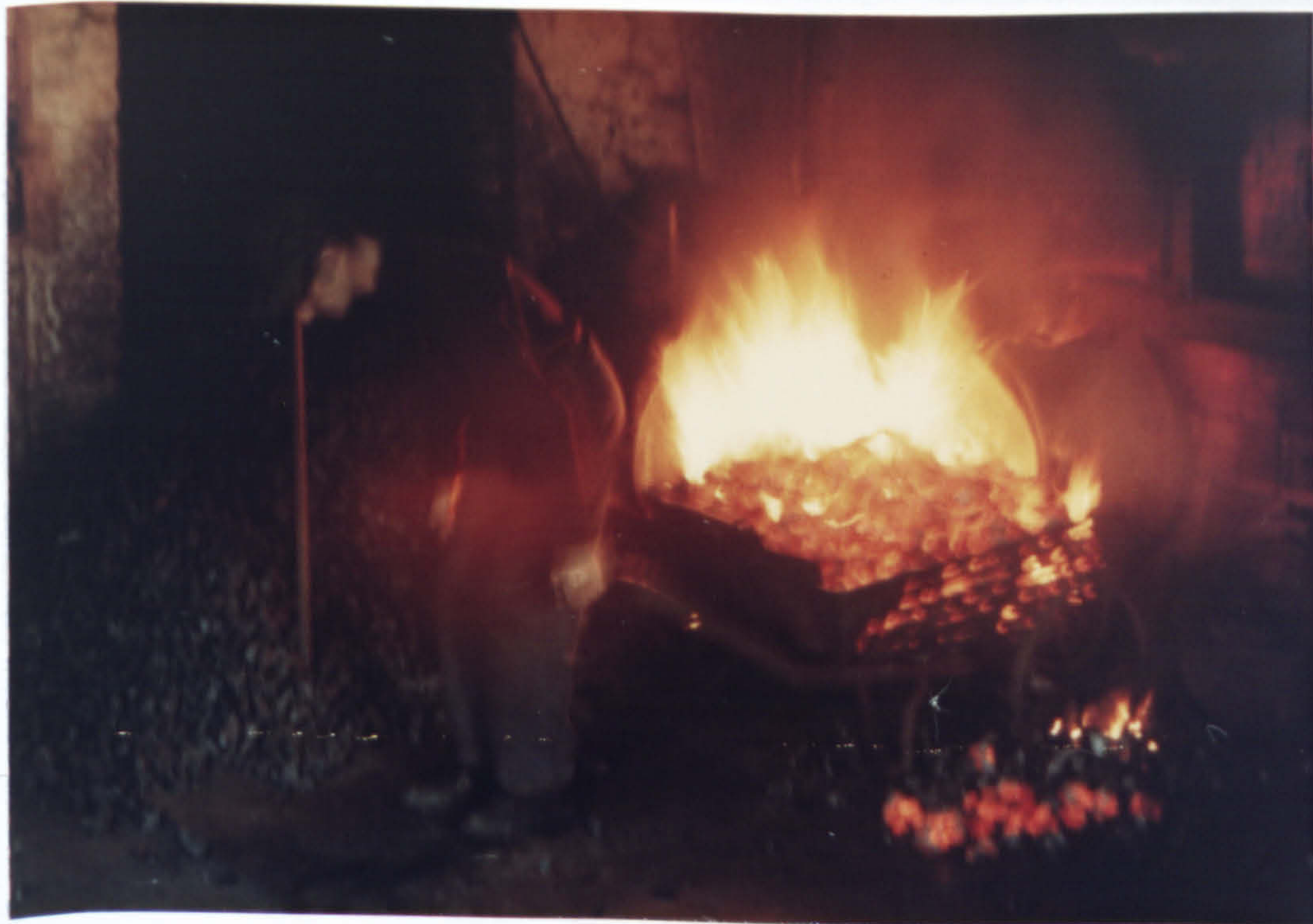
Removal of coke-barrow to water-quench outside retort house.
