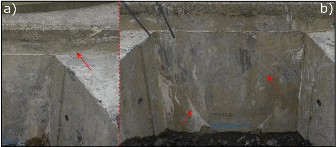
Figure 6.4: Physical appearance of a) “Initiation” cracks at the rib-plinth interface and b) “Propagation” face cracks with “U” shape form.
