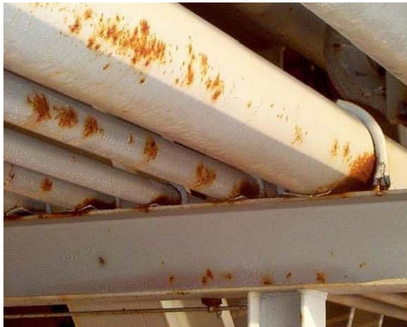
Figure 2.3: Example of corrosion at pipe supports 2
