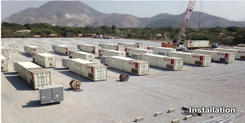
Figure 2: Battery-based energy storage systems (APR Energy, 2018).
