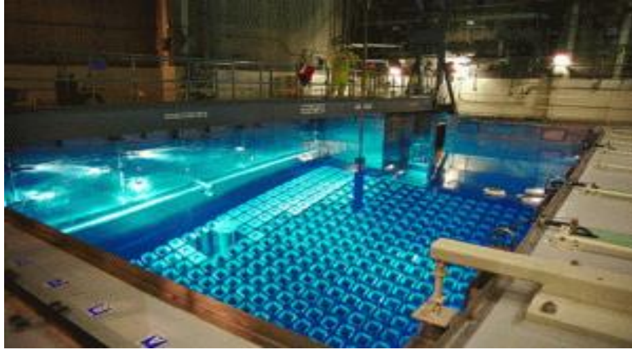
Figure 5: Bars or nuclear fuel in nuclear reactor (water being used as cooling fluid) (ANS Nuclear Cafe, 2014).
