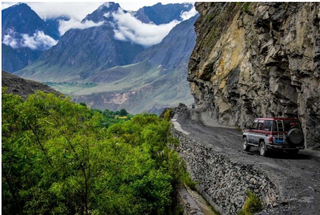
Figure 4.6: Road near Ayan Pic 2018 Courtesy of FT
