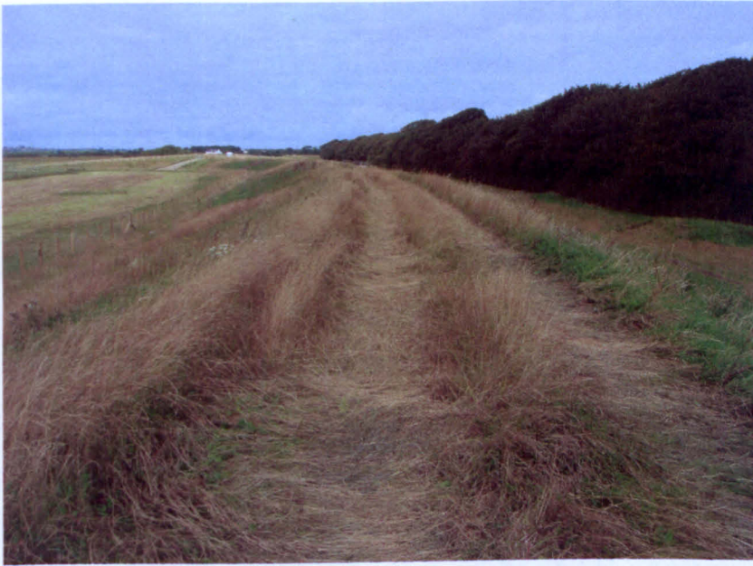
Figure 3.36 Flood embankment along River Lune, Lancaster.
