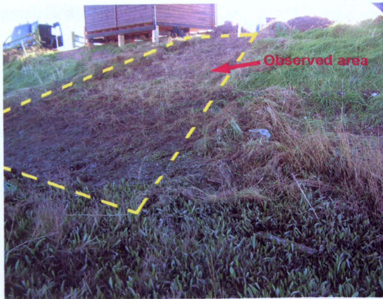
Figure 3.21 Observed area along the inland side embankment.
