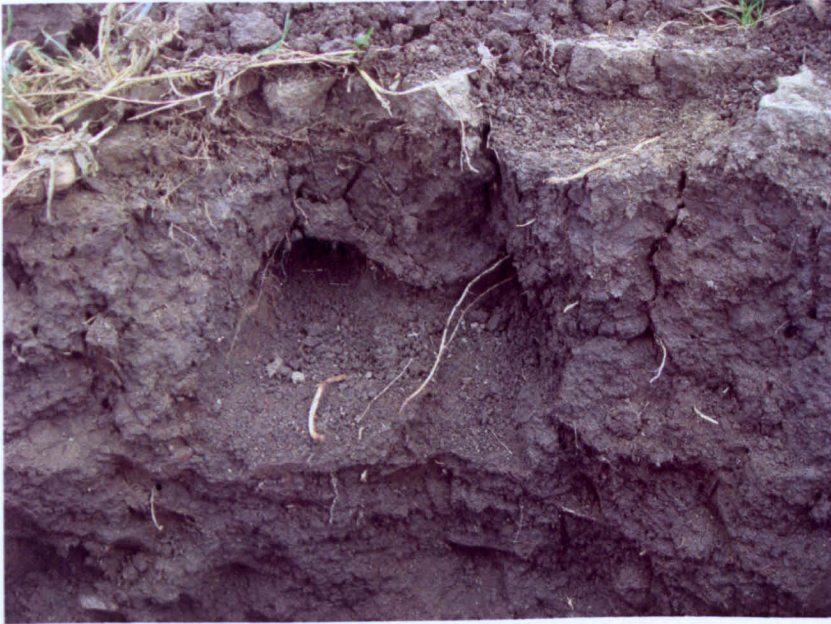
Figure 3.27 Animal burrowing close to the crest surface.
