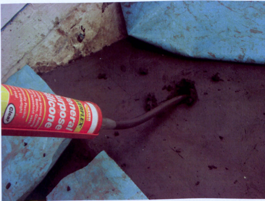
Figure 5.22 Injection of the slurry paste using silicone gun and flexible pipe.
