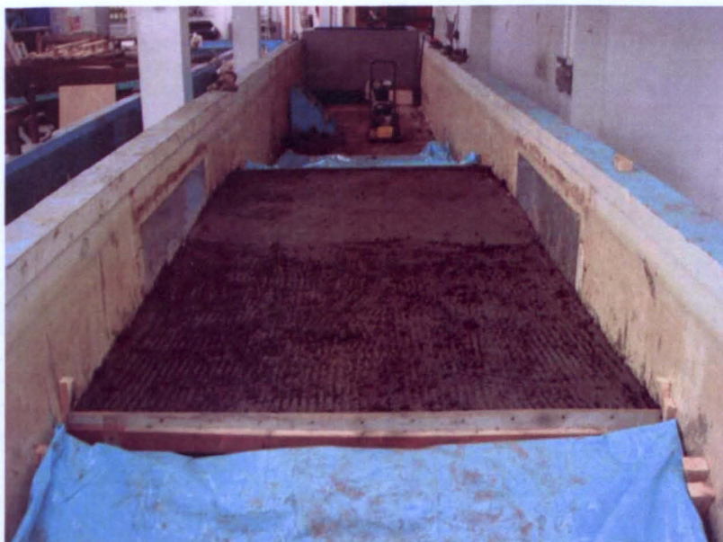
Figure 4.21 Scraped surface prepared for the next layer placing.
