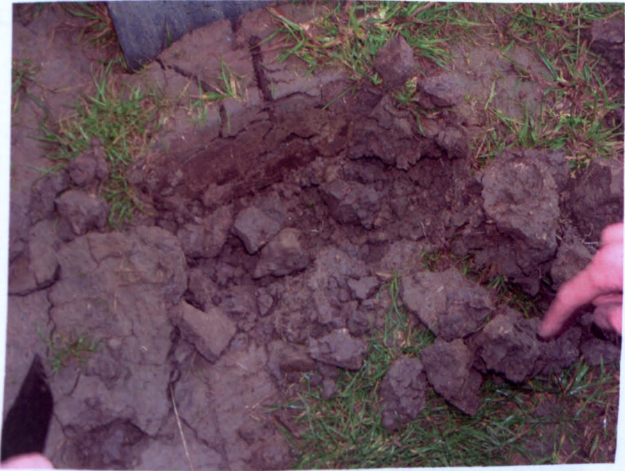
Figure 14.8 Hand excavation on the new embankment.
