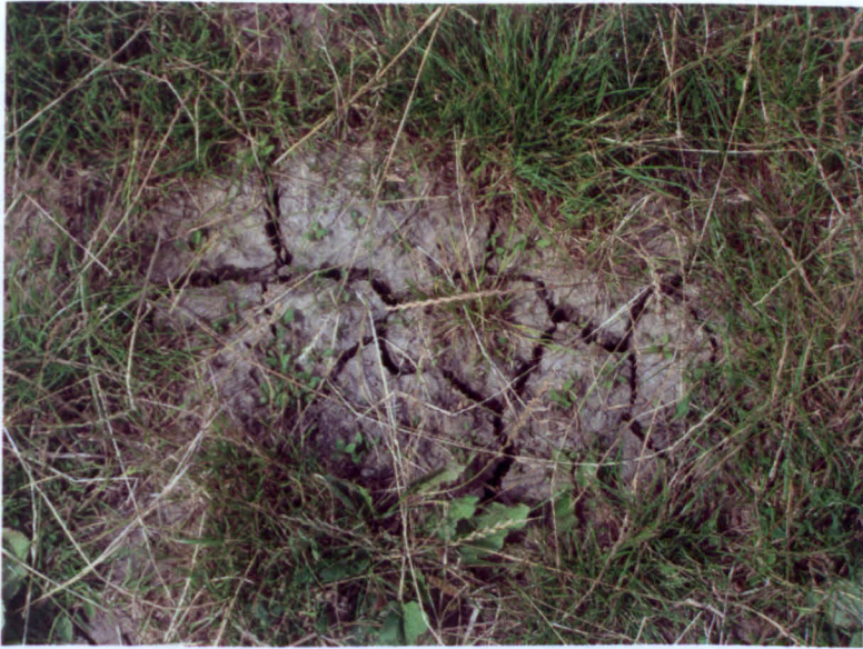
Figure 3.25 Desiccation cracking observed in York.
