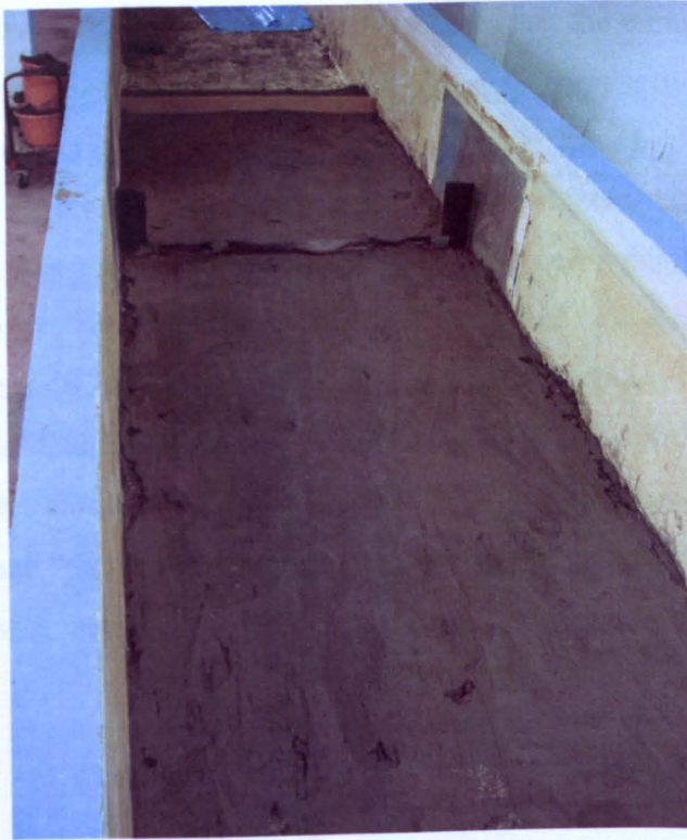
Figure 4.17 Berm compacted to desired state.
