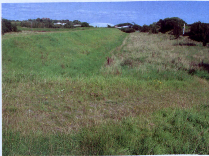
Figure 3.30 Embankment along reservoir, Bridport.
