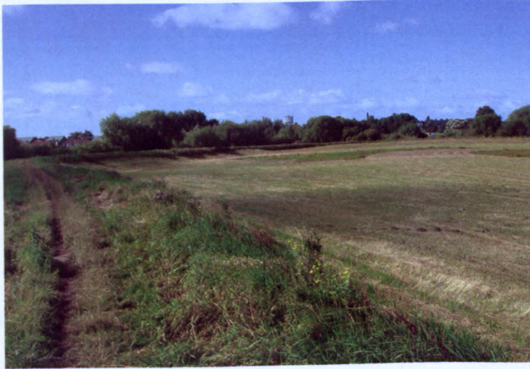
Figure 3.23 Embankment along River Ouse.
