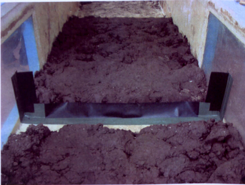
Figure 4.16 Installed cut-off barrier.
