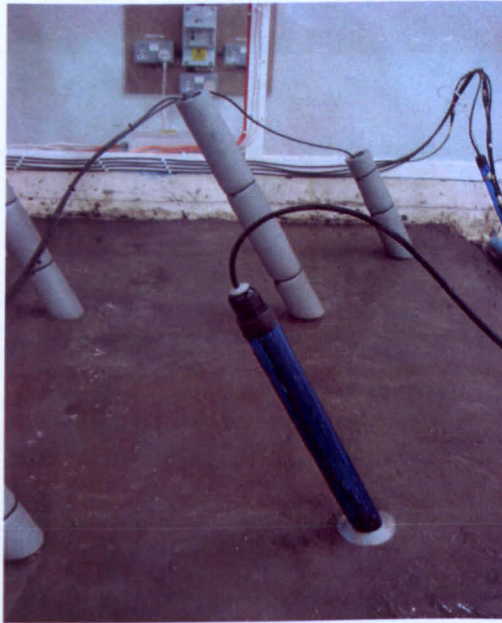
Figure 5.28 Tensiometers protected by insulation.
