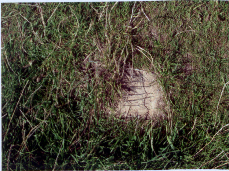
Figure 3.32 Desiccation cracking observed at Bridport embankment.
