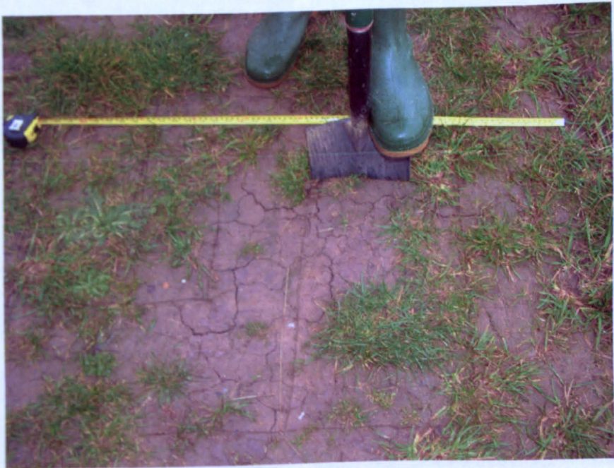
Figure 14.7 Hand excavation on the new embankment.
