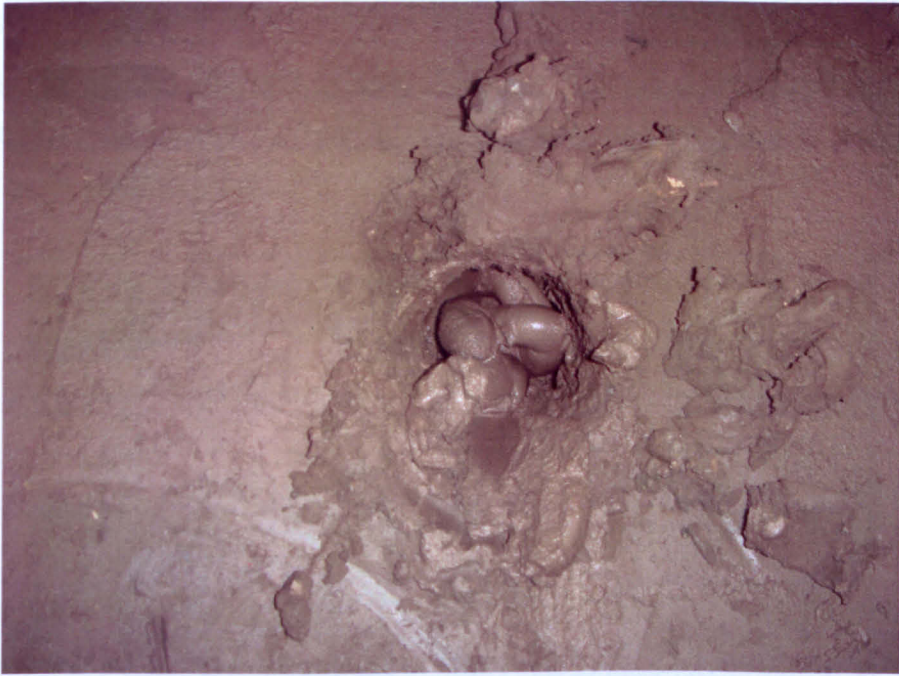
Figure 5.23 Slurry paste inside the hole.
