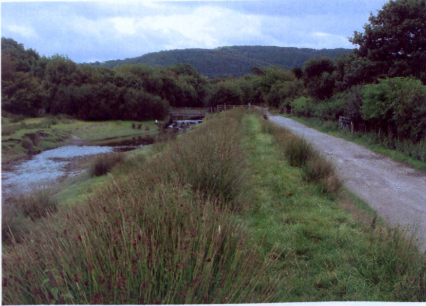
Figure 3.33 Embankment along River Resr.
