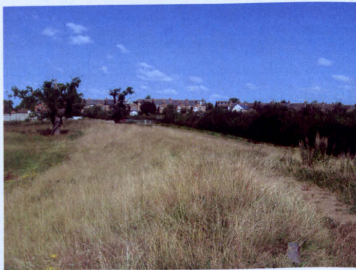
Figure 3.28 Embankment along Thames River at Windsor.
