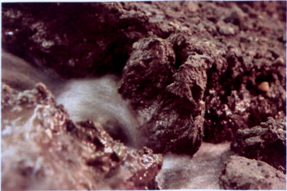
Figure 8.23 Pushed away clay block.
