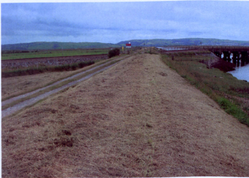
Figure 3.34 Embankment along Dovey estuary, Gwynedd.
