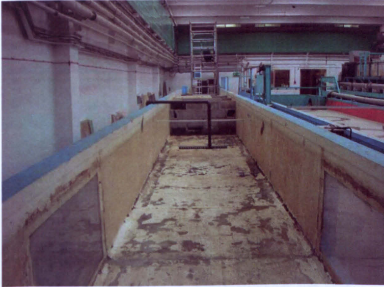
Figure 4.15 Concrete flume with diffuser and windows where the model was constructed.
