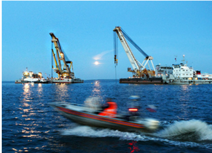
Figure 1: Floating Cranes for marine salvage [61]
