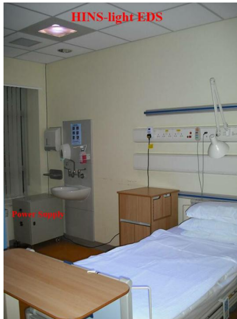
Fig. 7.1. HINS-light Environmental Decontamination System (HINS-light EDS) in a hospital isolation room (Glasgow Royal Infirmary, Scotland, UK).
