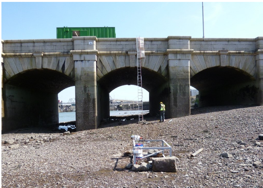
Figure 5.4: Test arrangement viewed from the seabed
