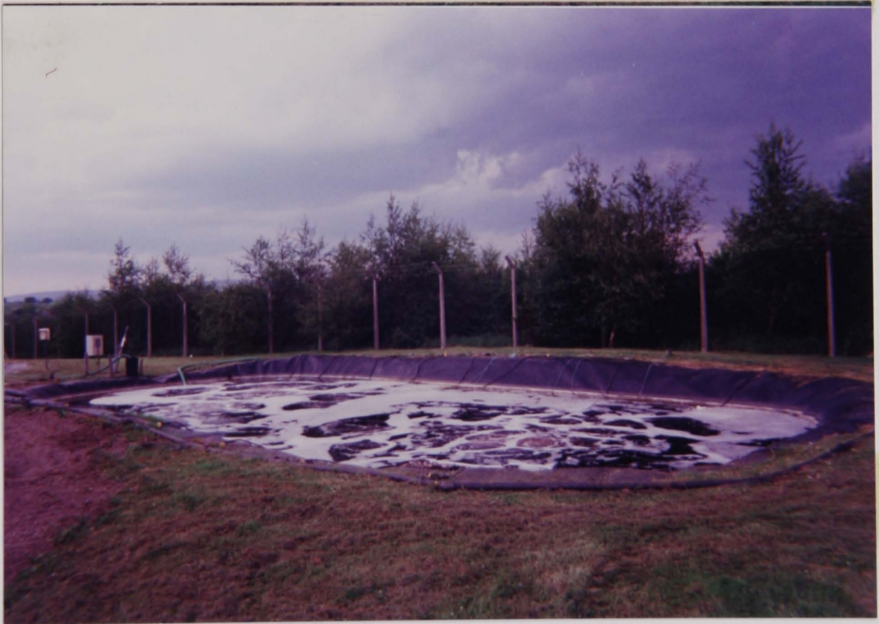
Figure 5.9 On Site Leachate Treatment Pond II
