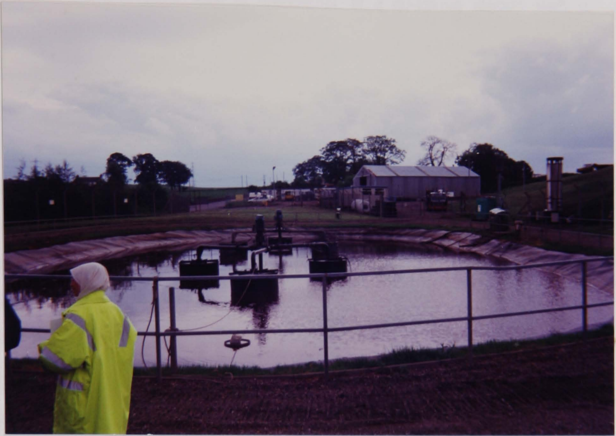
Figure 5.8 On Site Leachate Treatment Pond I
