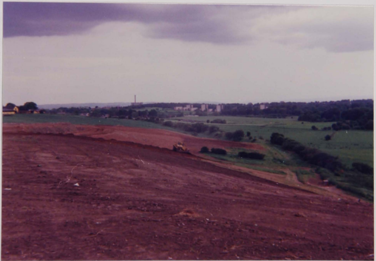
Figure 5.11 Restored Landfill Site
