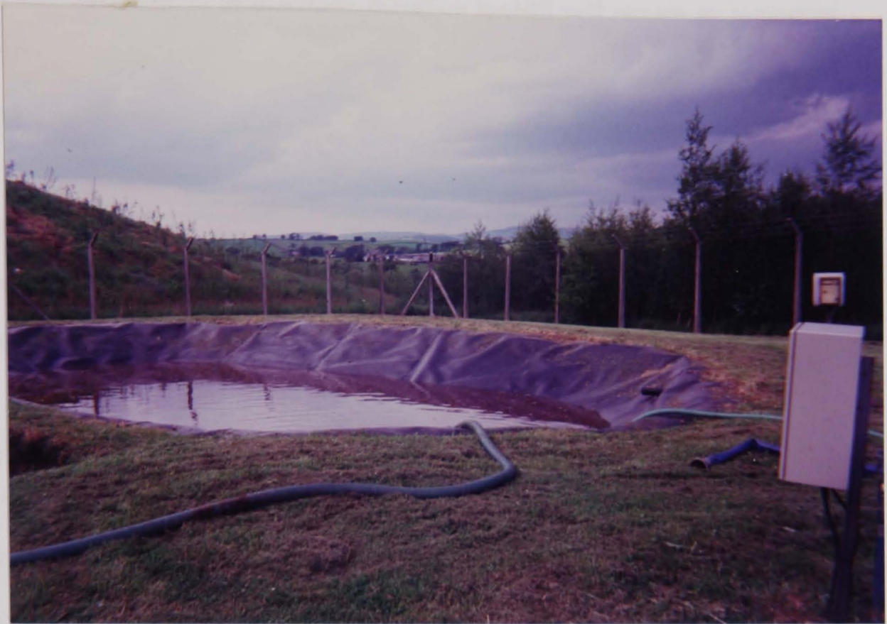
Figure 5.10 On Site Leachate Treatment Pond III
